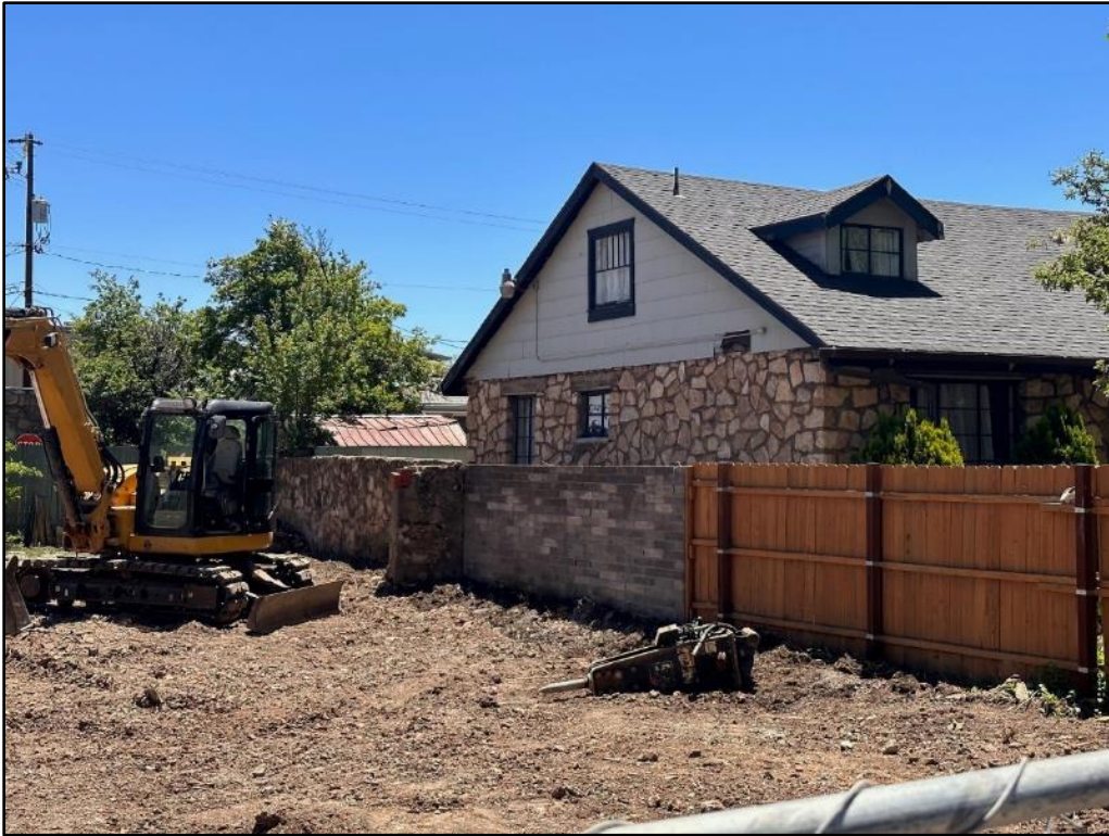
Plate 4. View southeast toward north elevation.
