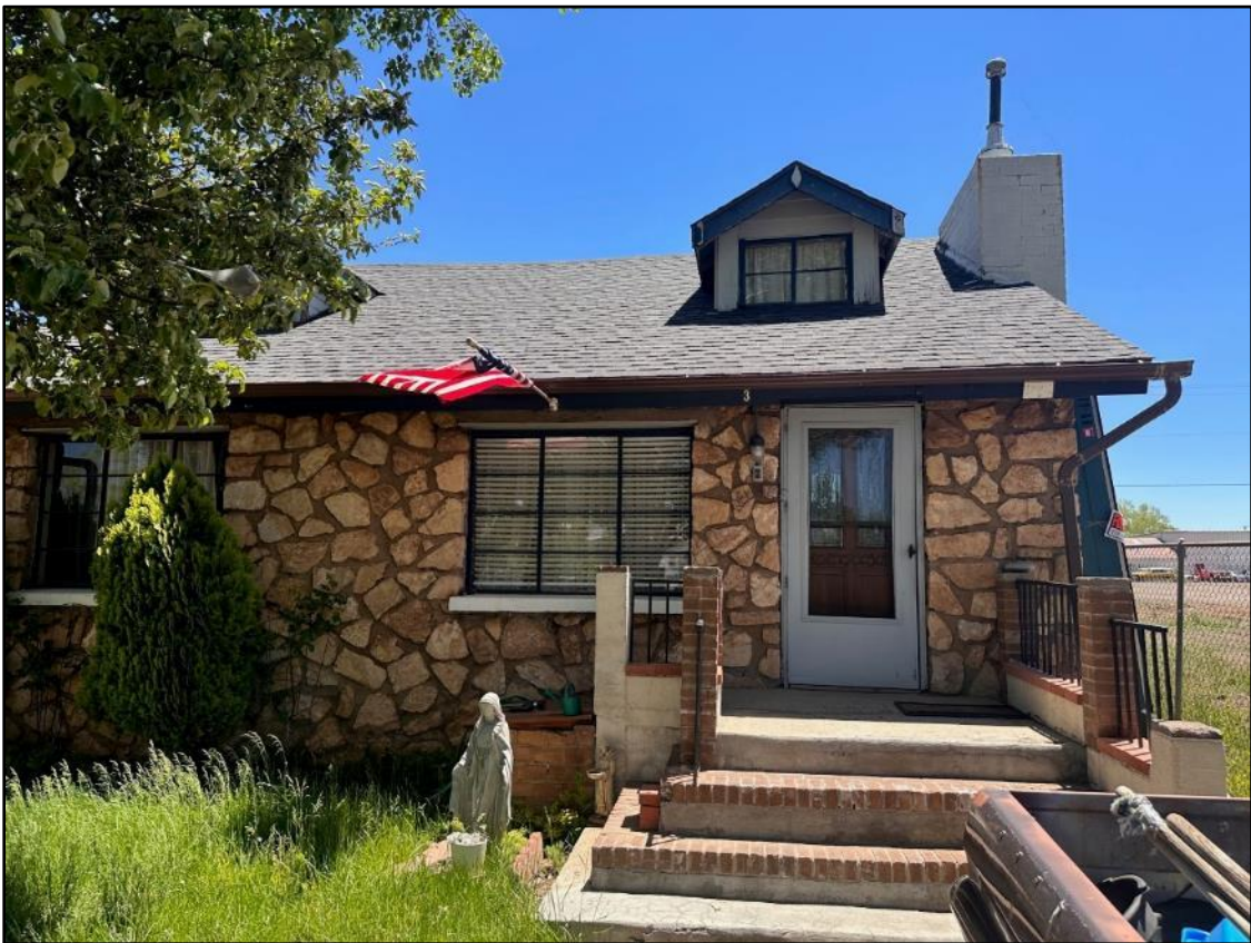
Plate 2. View east toward main entrance of west façade.
