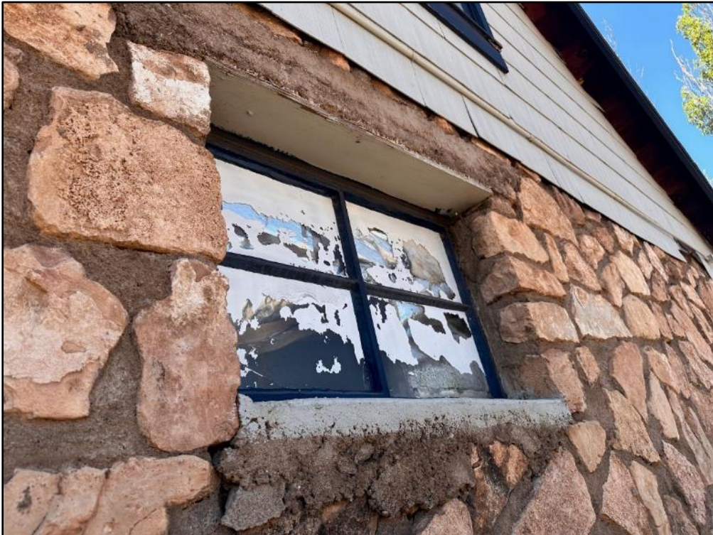
Plate 7. View of north elevation window.
