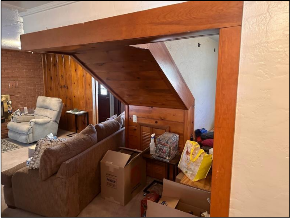
Plate 13. View of living room toward front entry, showing stairway finish.
