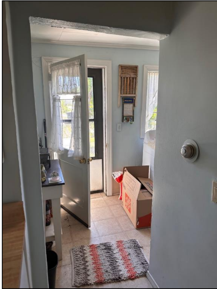
Plate 23. View of rear ell entry/laundry area.
