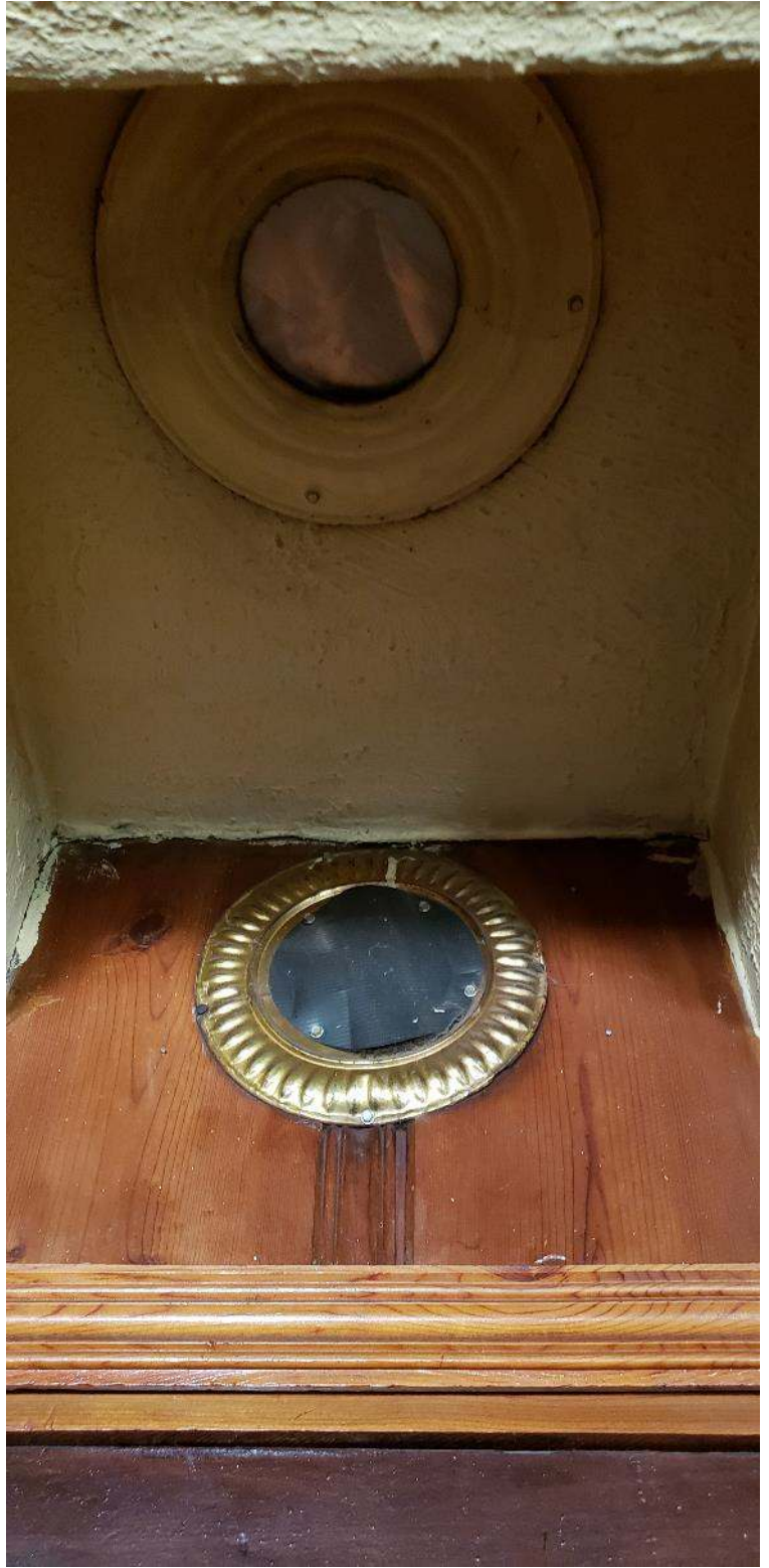
Photos 33–34. 617 W Tombstone back of house SW corner bedroom and laundry room from SE corner room facing W (left) and detail of where a stove pipe once went outside through the house's S façade and the roof, facing S/up (right); the latter photo is evidence of the back room likely being added on at some point.
