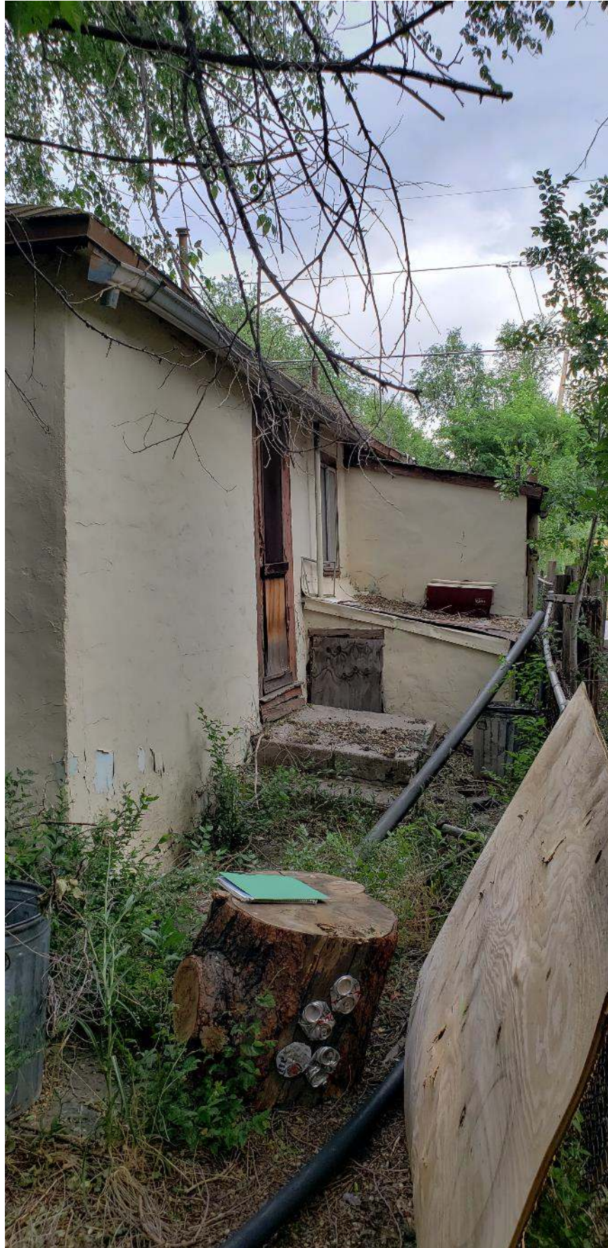
Photo 11. 617 W Tombstone Ave E façade at SE corner to N.
