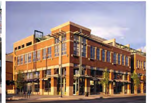
Parking areas should be screened from public view. When facing a public street, design the edges with active building uses, when feasible, or design to look like a building with similar bay rhythm and materiality. When facing an alley, use creative screening techniques, such as mesh, screens, green walls, or design to look like a building.
