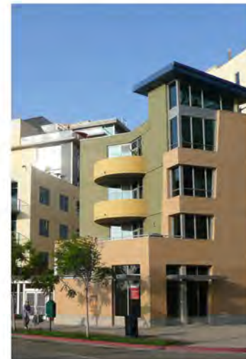
An eye-catching, mixed use building at the corner of Edgen and Route 66 could serve as a gateway to downtown.
