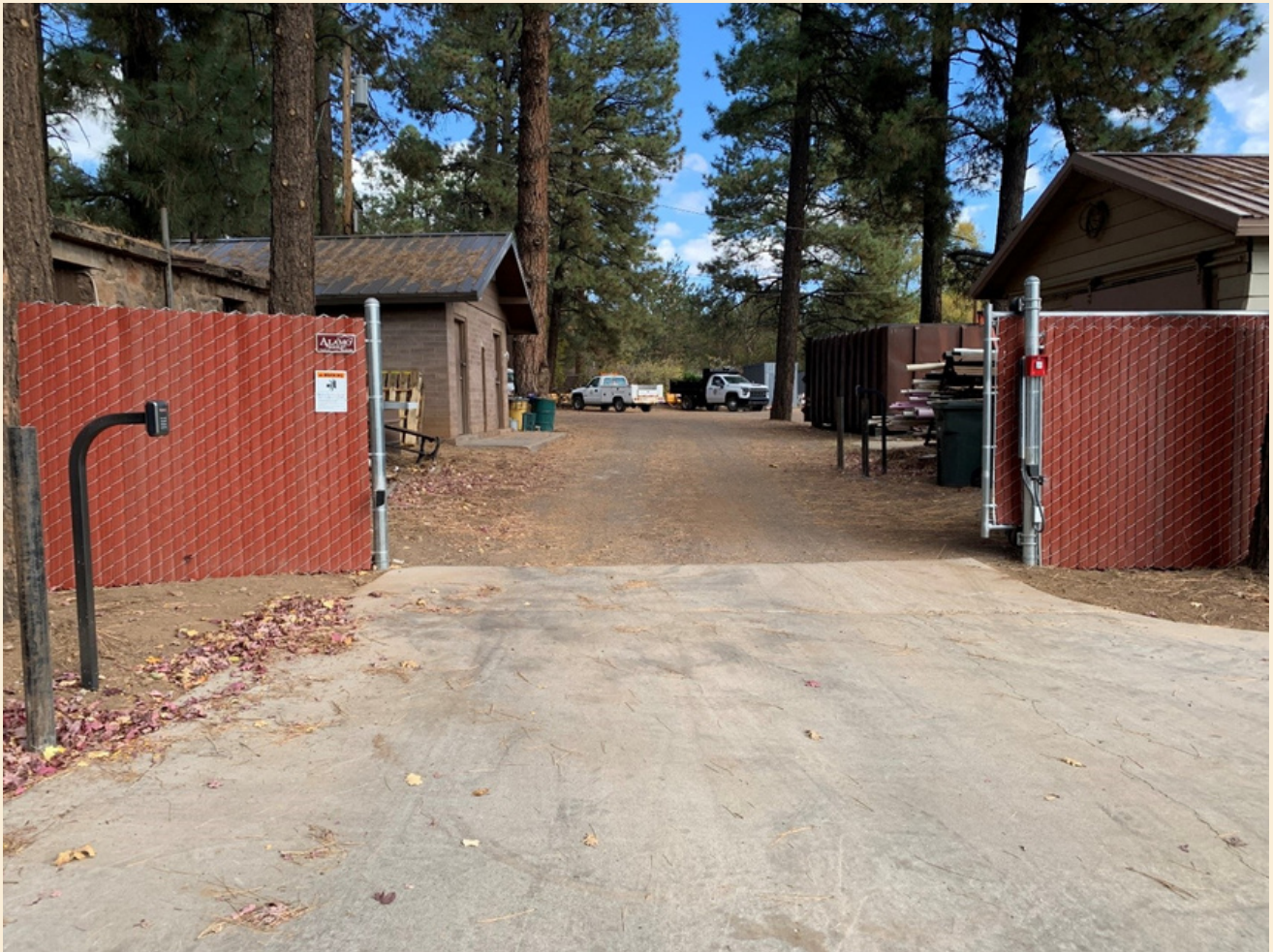
Above: The new automated gate.
