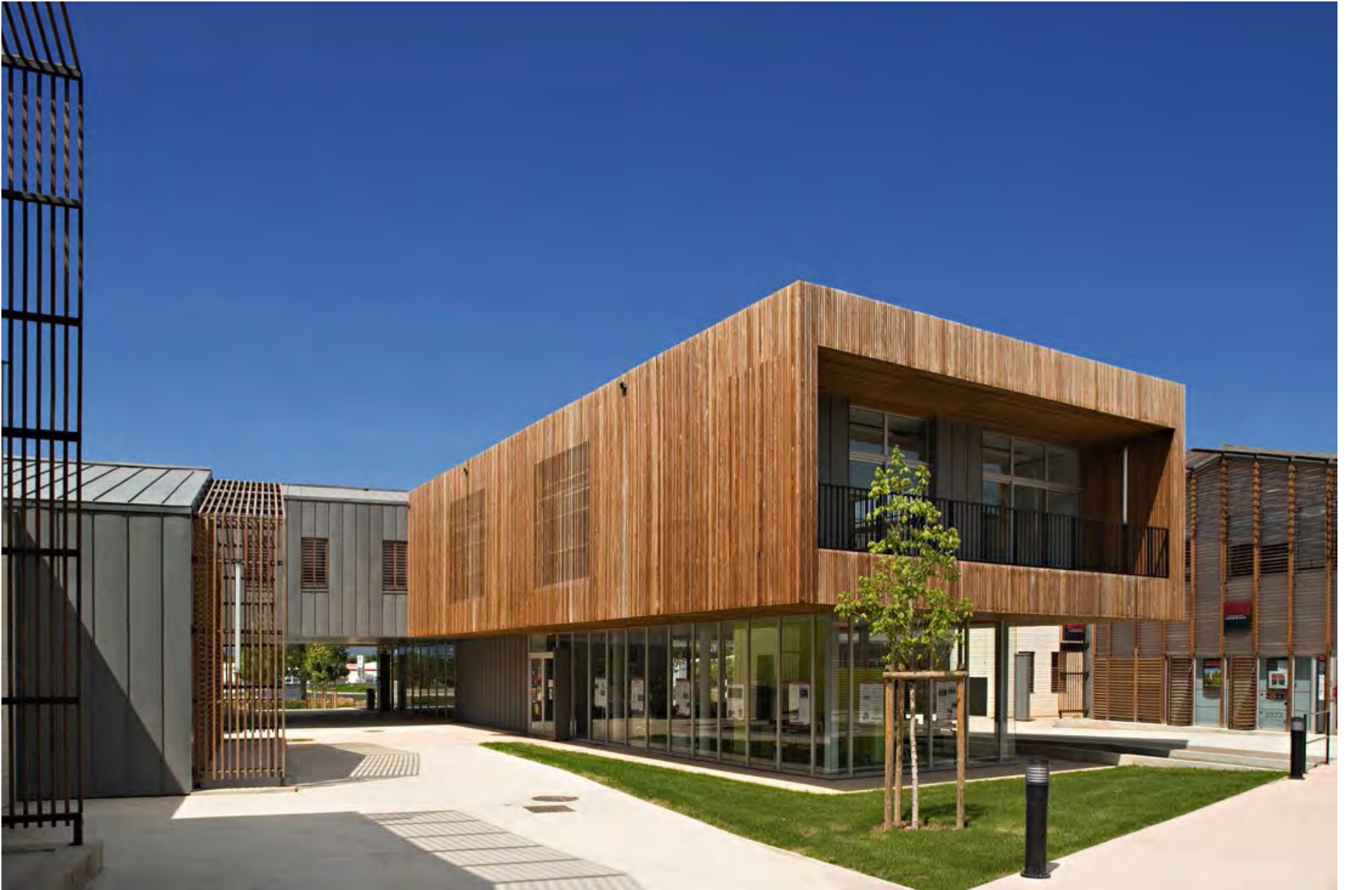
Image 52, Pre-patinaed metal, integrated window screening, outdoor balconies, and wood. Deep overhangs and extended vertical planes.
