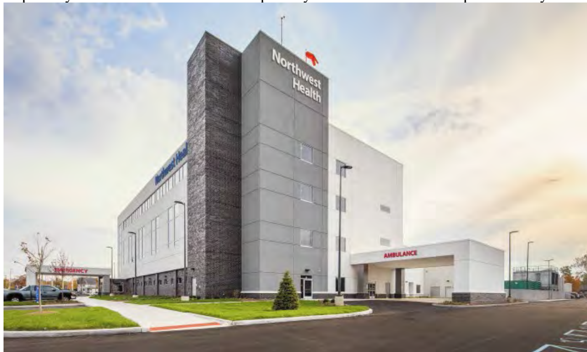
Image 57, EIFS as a primary material. EIFS forms define building elements and express articulation through different colors, scoring and texture.
