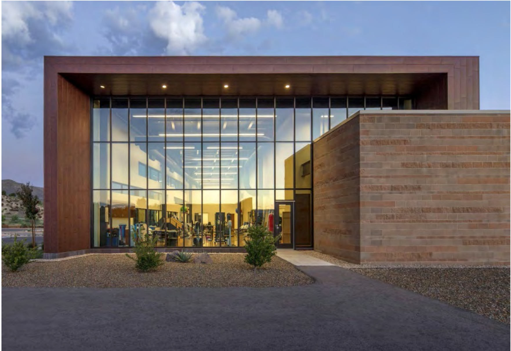
Image 50, Warm colored metal panels, textured masonry, dark window framing, deep horizontal and vertical projections.
