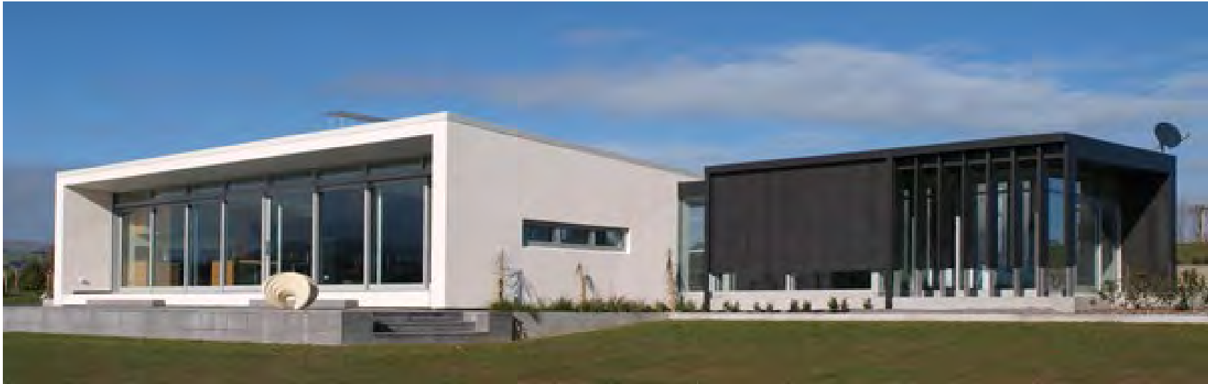
Image 56, EIFS as a primary material. EIFS forms define primary elevations and are complimented by other building materials.
