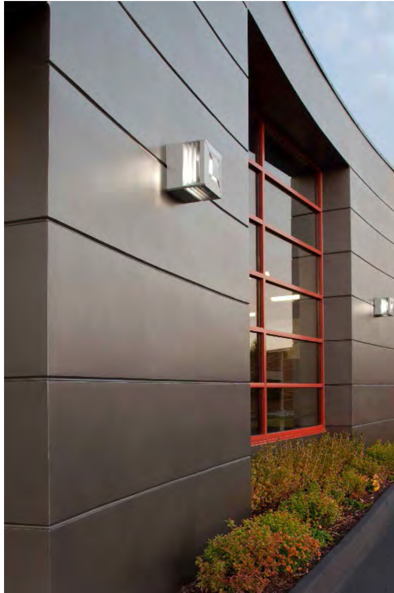
Image 59, EIFS as a primary material. EIFS used to express unique façade textures and provide reference to alternate materials.
