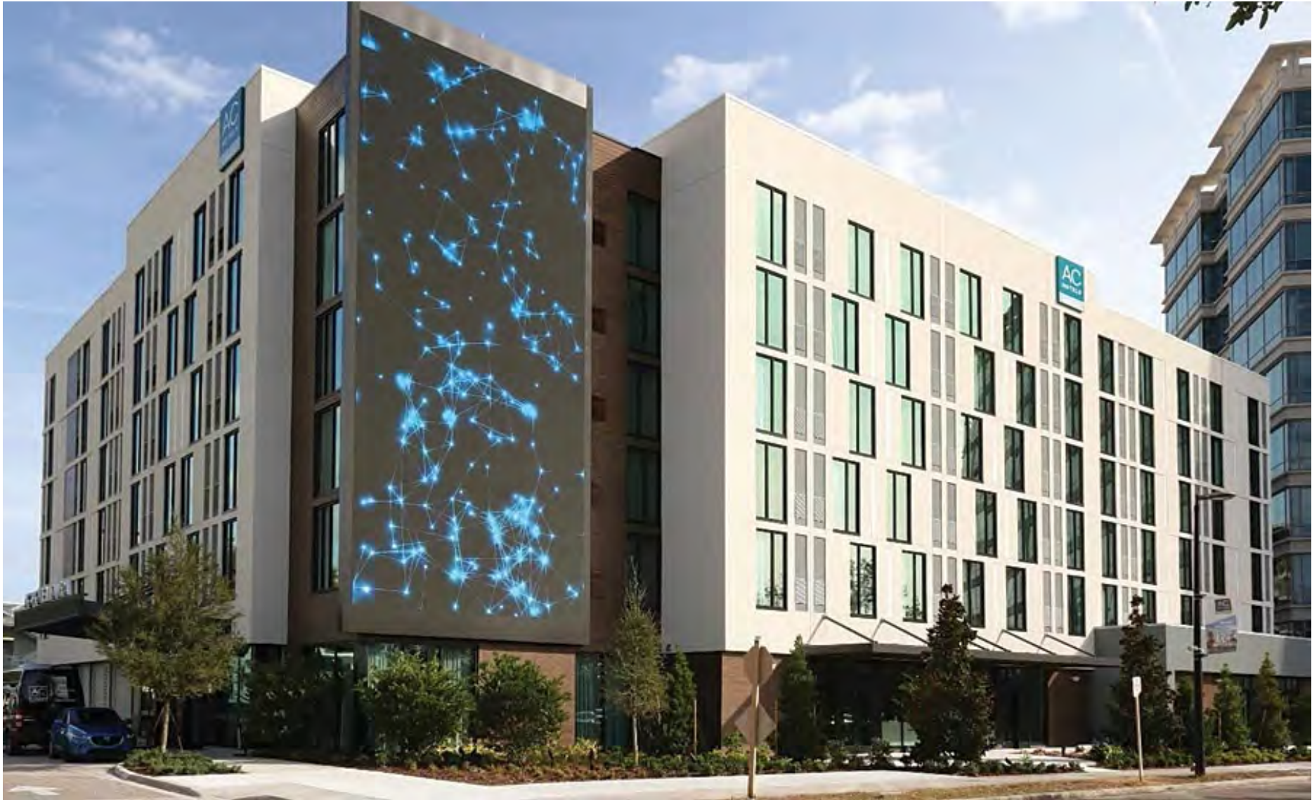
Image 58, EIFS as a primary material. EIFS forms provide a modern façade treatment at a larger scale.
