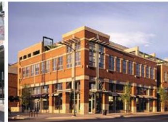
Parking areas should be screened from public view. When facing a public street, design the edges with active building uses, when feasible, or design to look like a building with similar bay rhythm and materiality. When facing an alley, use creative screening techniques, such as mesh, screens, green walls, or design to look like a building.
