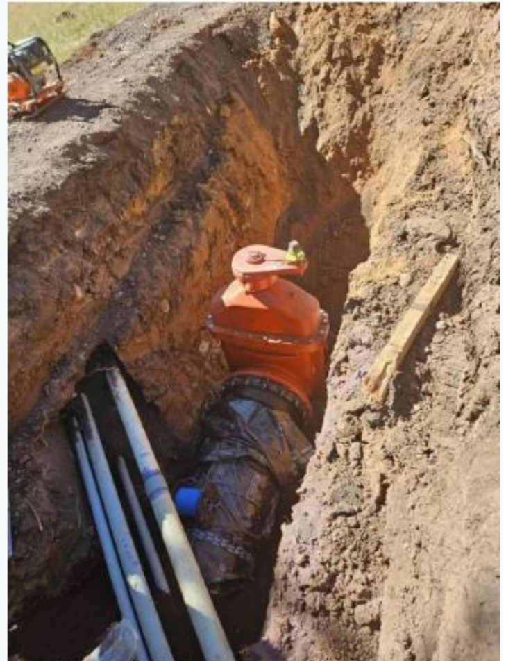
Installation of the 24" ductile iron water transmission main
