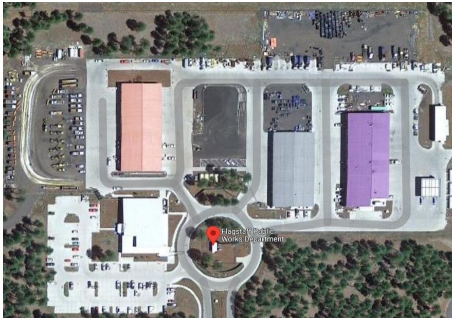
Figure 3-4. Public Works Department Facility
