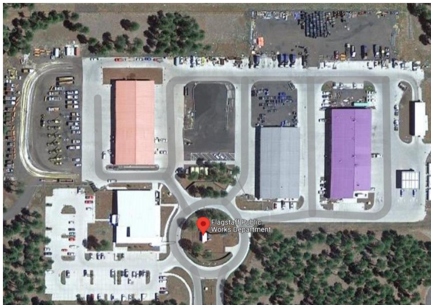
Figure 3-4. Public Works Department Facility
