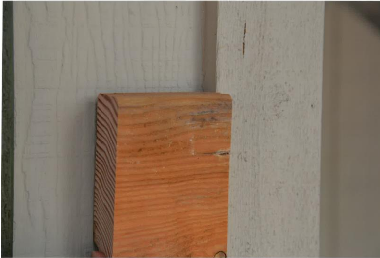
Window + door strips to be trimmed with \frac{1}{2} " thicker wood to accommodate clapping.
