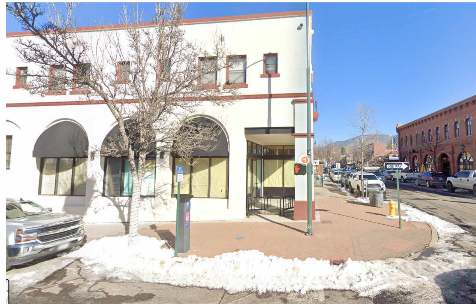
EXISTING VIEW FROM W ASPEN AVE
