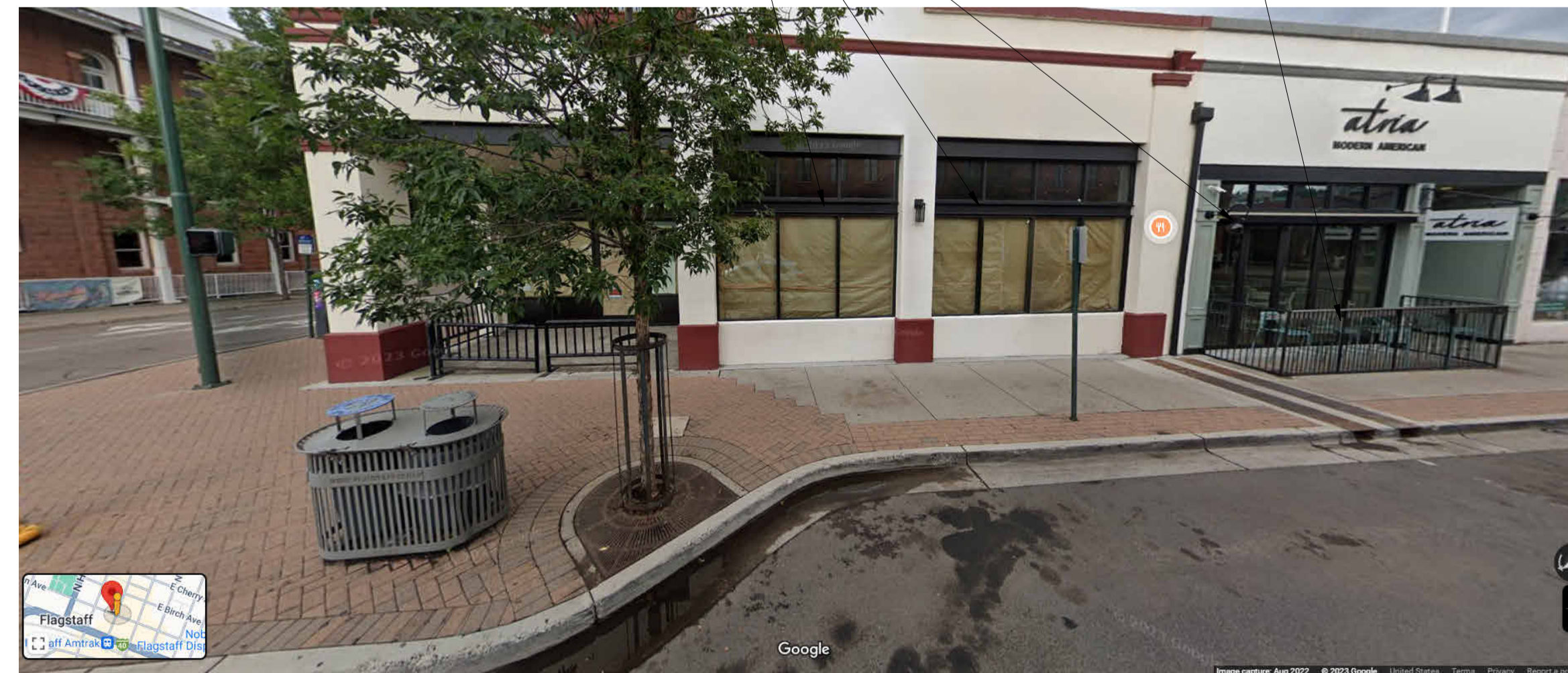
EXISTING VIEW FROM N LEROUX ST
