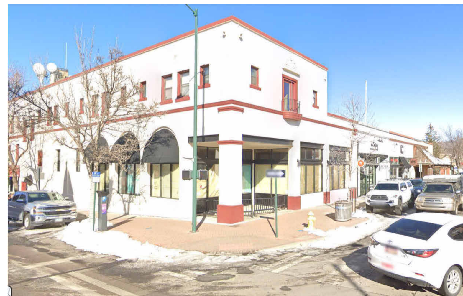
EXISTING VIEW FROM CORNER
