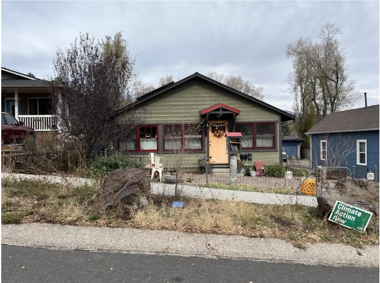
Photo 1. 810 West Grand Canyon Avenue. Photo facing north-northwest.
