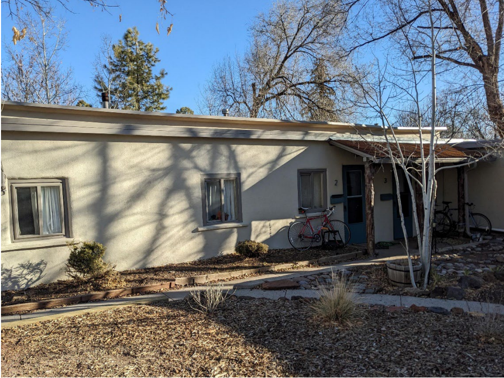
Completed stucco, wood and roof work at 823 W Aspen Ave
