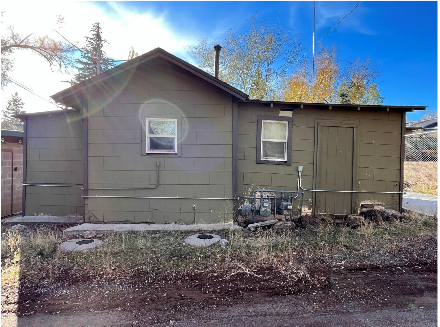
Photo 3. Rear (north) facade of 810 1/2 West Grand Canyon Avenue. Photo facing south-southeast.
