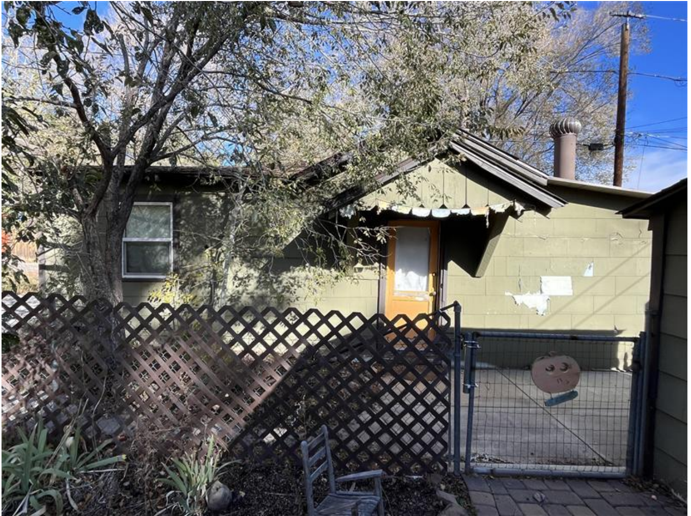
Photo 2. Primary facade of 810 1/2 West Grand Canyon Avenue. Photo facing north-northwest.
