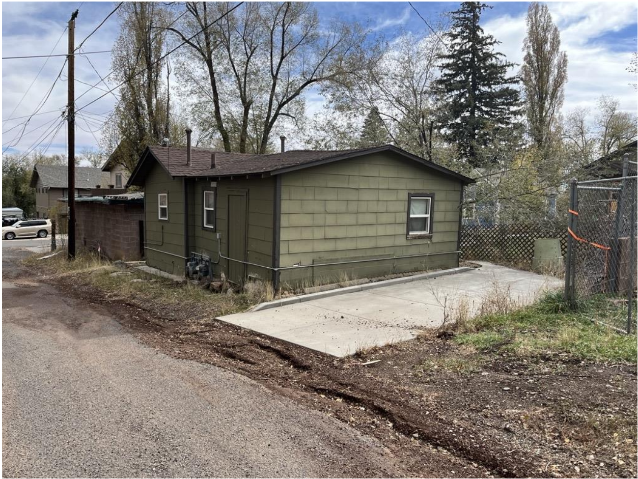
Photo 6. Overview of 810 1/2 West Grand Canyon Avenue. Photo facing southeast.
