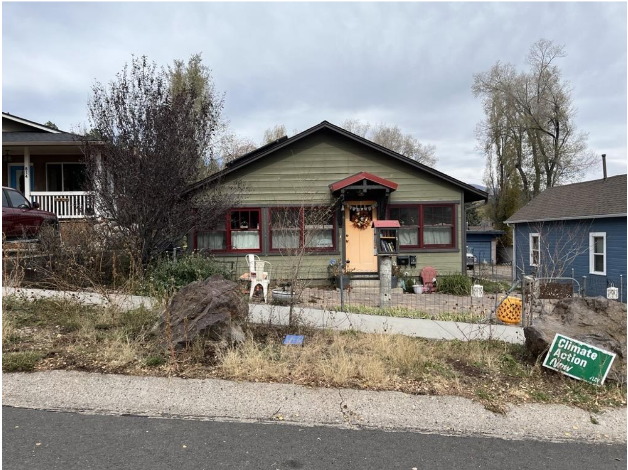
Photo 1. 810 West Grand Canyon Avenue. Photo facing north-northwest.
