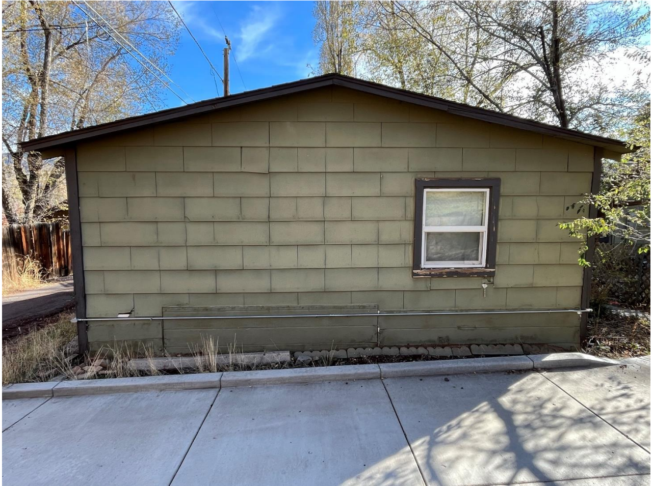
Photo 4. West (side) facade of 810 1/2 West Grand Canyon Avenue. Photo facing east.
