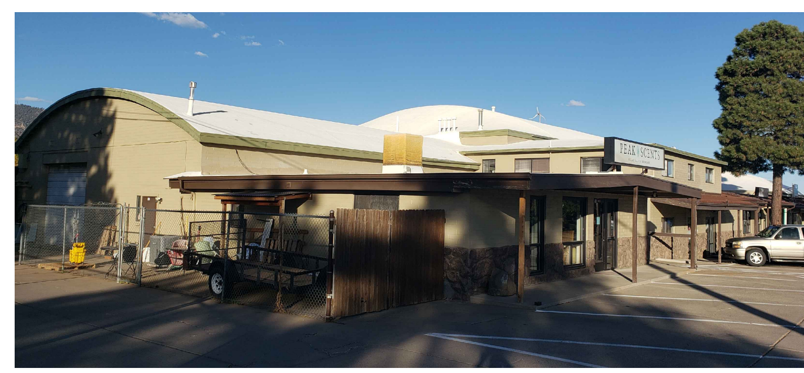
3 A2.1 PHOTO OF EXISTING BUILDING - WEST FACING
