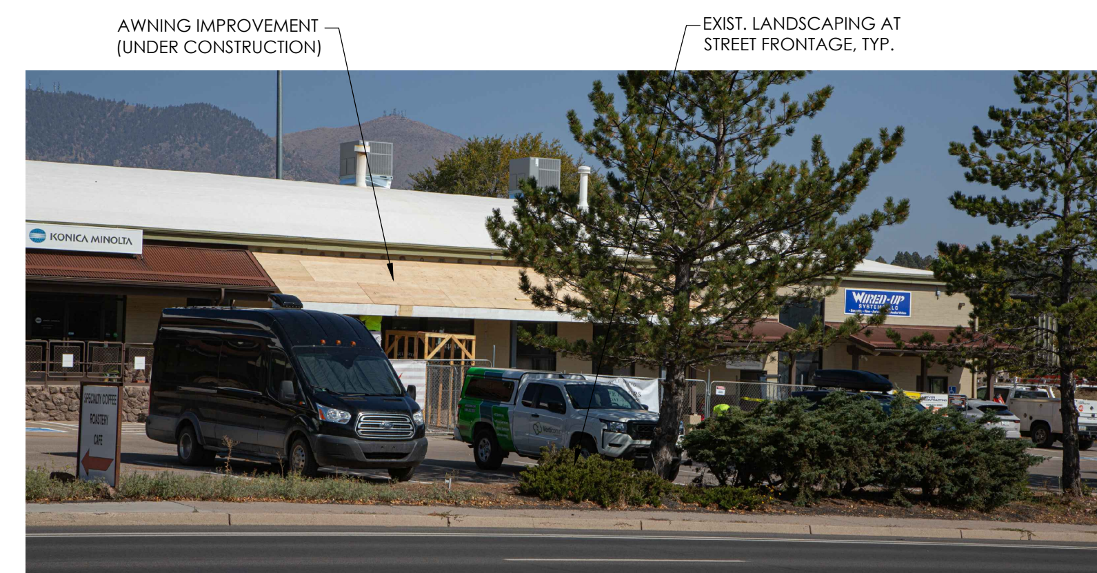
6 A2.1 PHOTO OF BUILDING IMPROVEMENTS (UNDER CONSTRUCTION)
