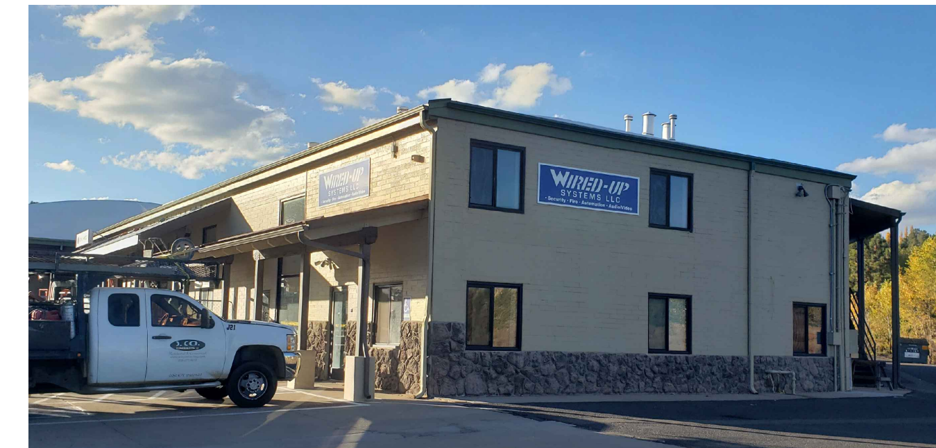
2 A2.1 PHOTO OF EXISTING BUILDING - EAST FACING
