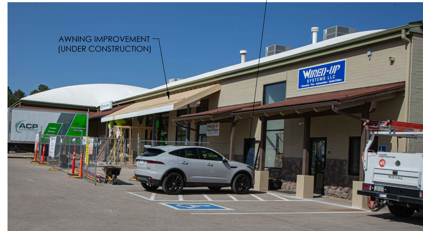
5 A2.1 PHOTO OF BUILDING IMPROVEMENTS (UNDER CONSTRUCTION)
