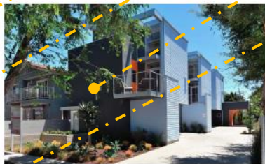
Small-lot Single-family Homes, Each on its Own Lot. Shared Driveway and Utility Easements. Front Unit is Oriented to the Street with Front Entrance and Path.
