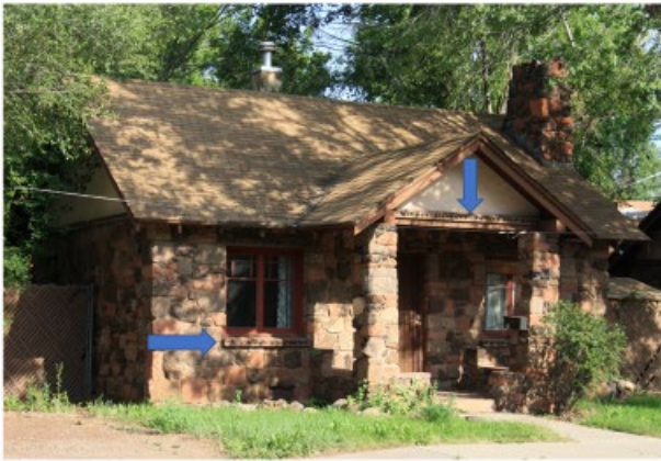
4 Square project stone houses prior to restoration. Note the decorative use of obsidian in concrete sills and lintels. Also the 1900s kitchen.
