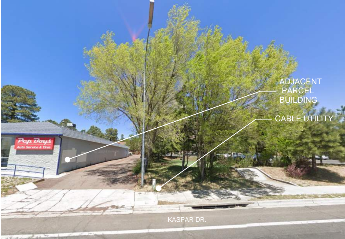
3. At West property line looking North
