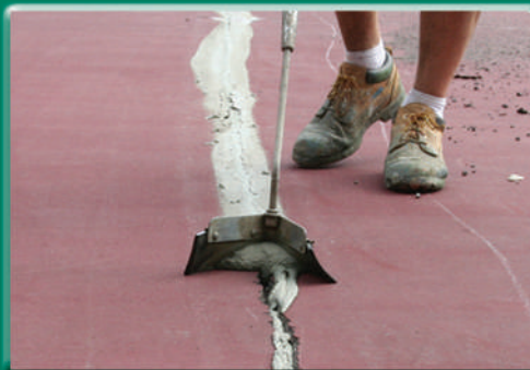
STEP 1: Fill cracks up to 4 inches wide
