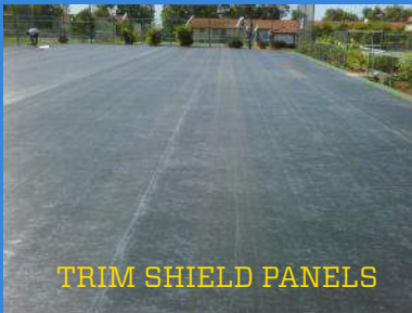
LAY THE SHIELD
