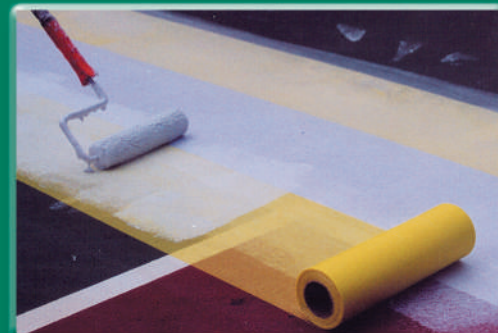
STEP 7: Install yellow ARMOR® mesh
