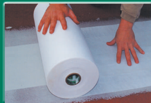
STEP 6: Install wide ARMOR® fabric
