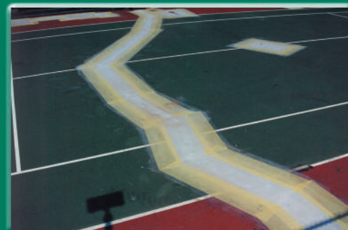
STEP 8: Finished...ready to color coat!
