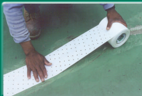
STEP 3: Apply ARMOR® release tape
