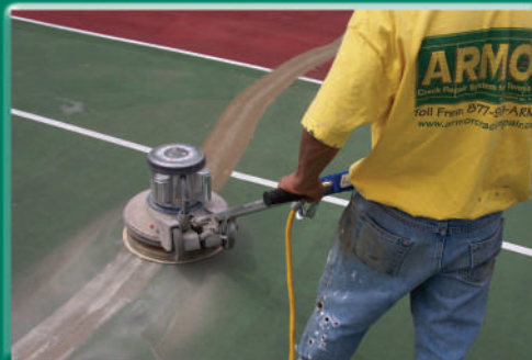
STEP 2: Sand flush to surface
