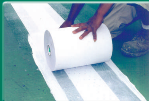
STEP 5: Install narrow ARMOR® fabric
