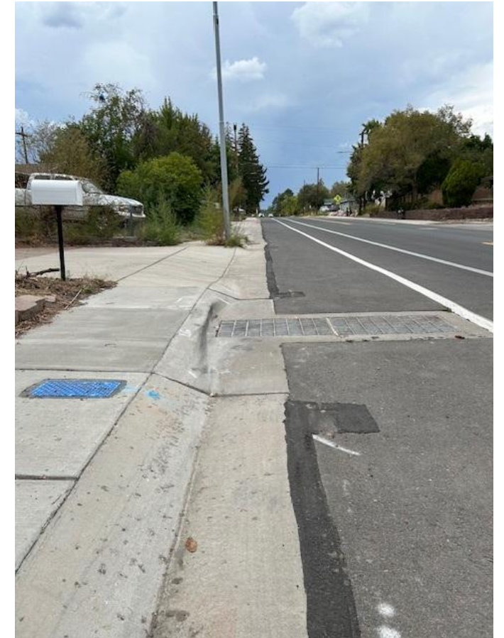
Finished trench with utility and stormwater crossings
