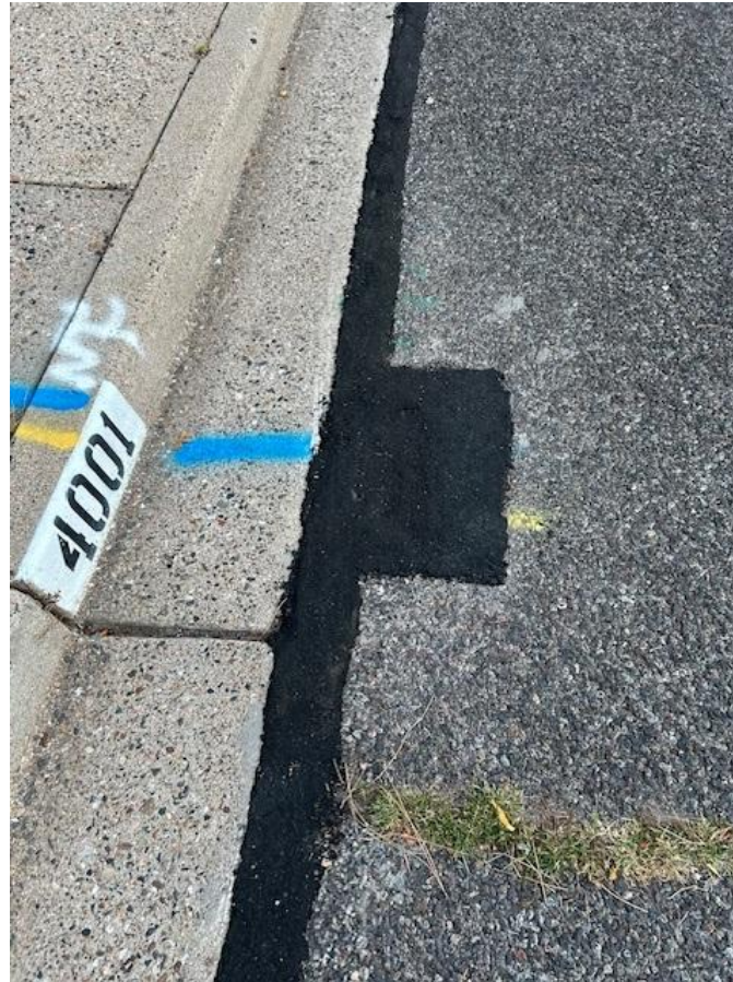
Finished trench with pothole patch at utility crossing
