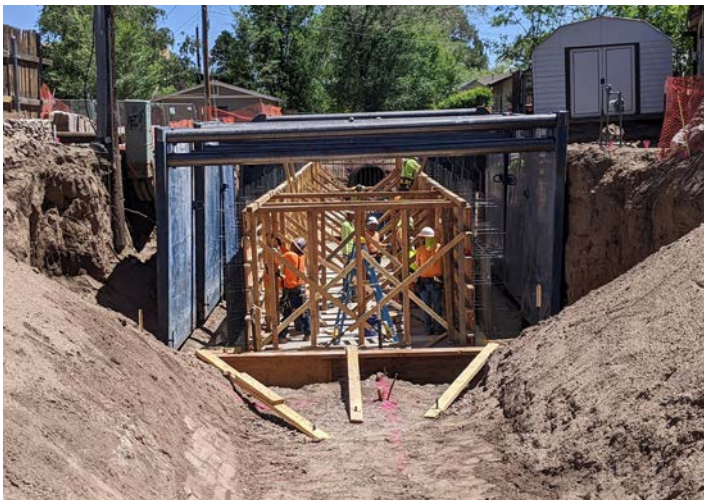
Drainage capital improvement.
