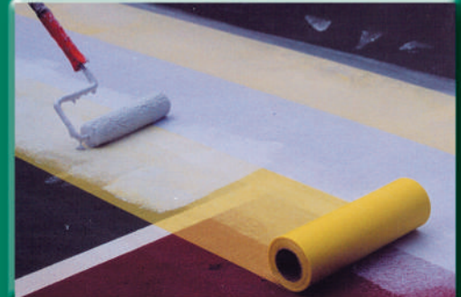
STEP 7: Install yellow ARMOR ® mesh
