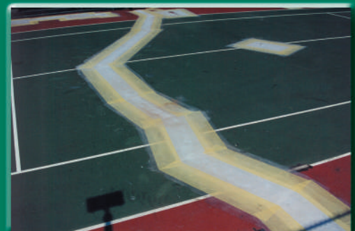
STEP 8: Finished...ready to color coat!
