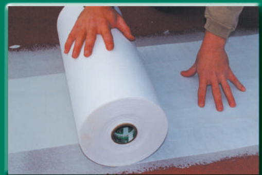
STEP 6: Install wide ARMOR ® fabric
