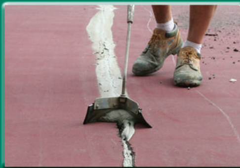
STEP 1: Fill cracks up to 4 inches wide
