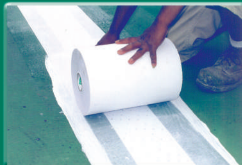
STEP 5: Install narrow ARMOR ® fabric
