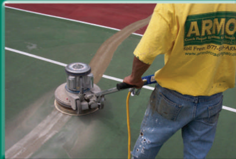
STEP 2: Sand flush to surface
