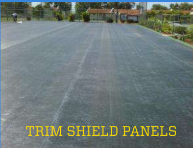
LAY THE SHIELD
