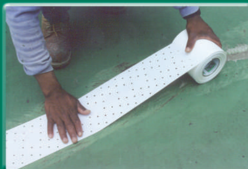
STEP 3: Apply ARMOR ® release tape
