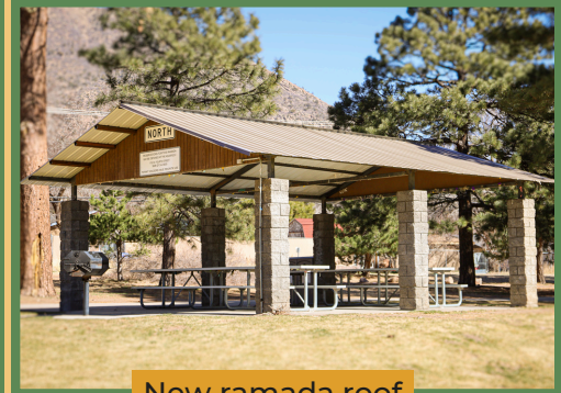
New ramada roof
