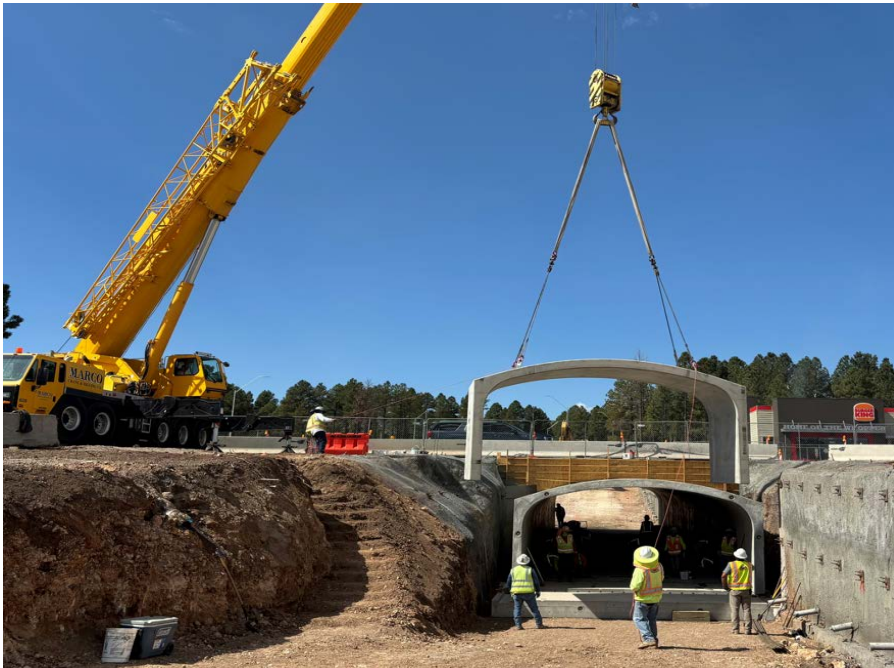
Pedestrian Tunnel Construction
