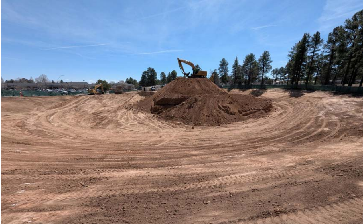
"The Wedge" Detention Basin
