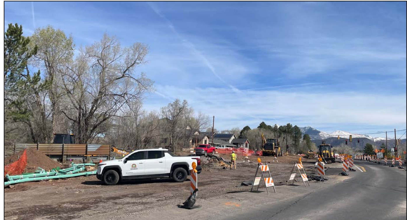
Lone Tree Corridor Inspection
