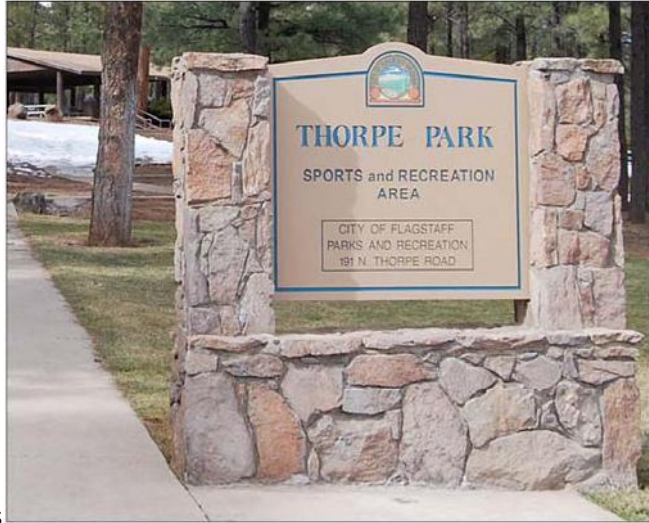
Sign Structure Materials
