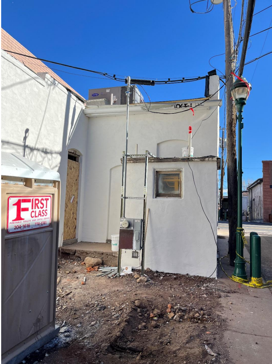
Photo of rear (West) elevation taken by author on December 27, 2024.
