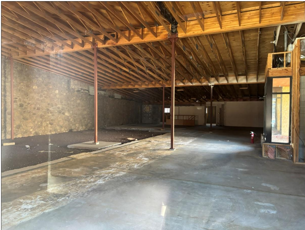
Photograph 5. The interior of 111 N Leroux Street, looking west, the original 1949 construction is located along the cinder area to the left. The southern wall of the building appears to be original and is shared with the neighboring building.
