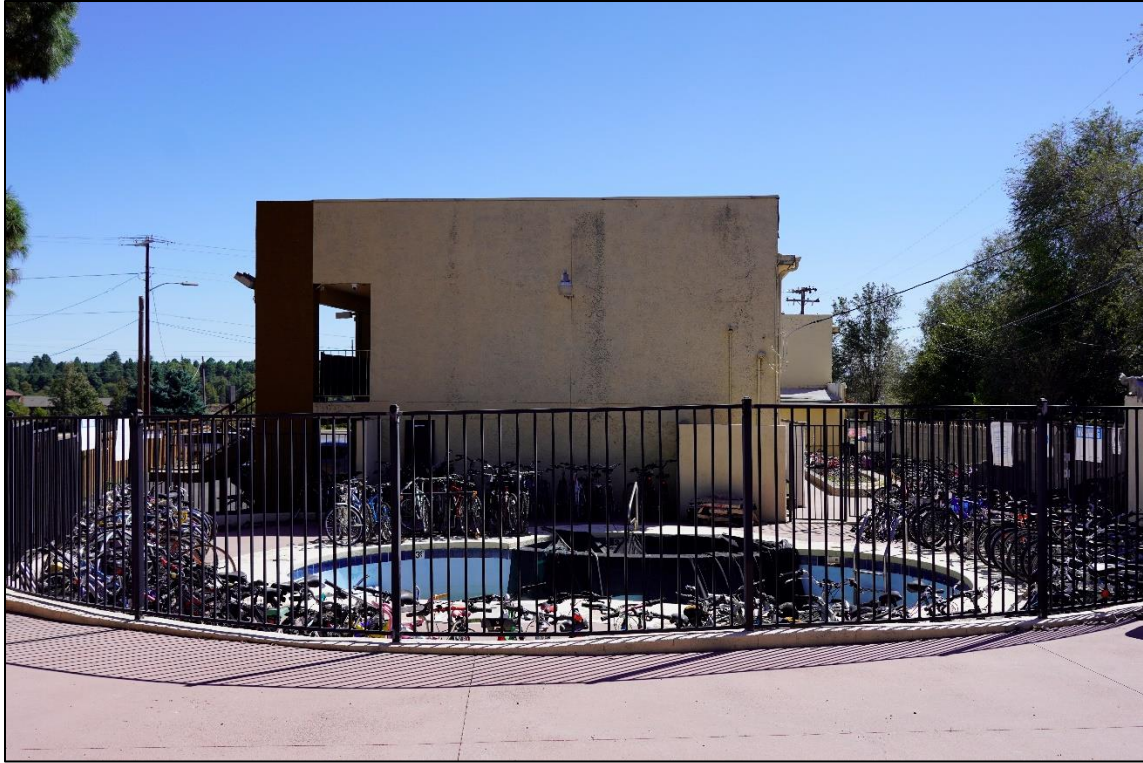
Figure 30. Photo of Building 2 and swimming pool, facing south.
