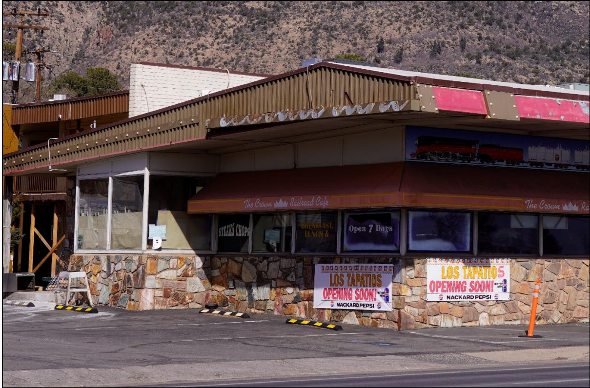
Figure 32. Photo of stone cladding.
