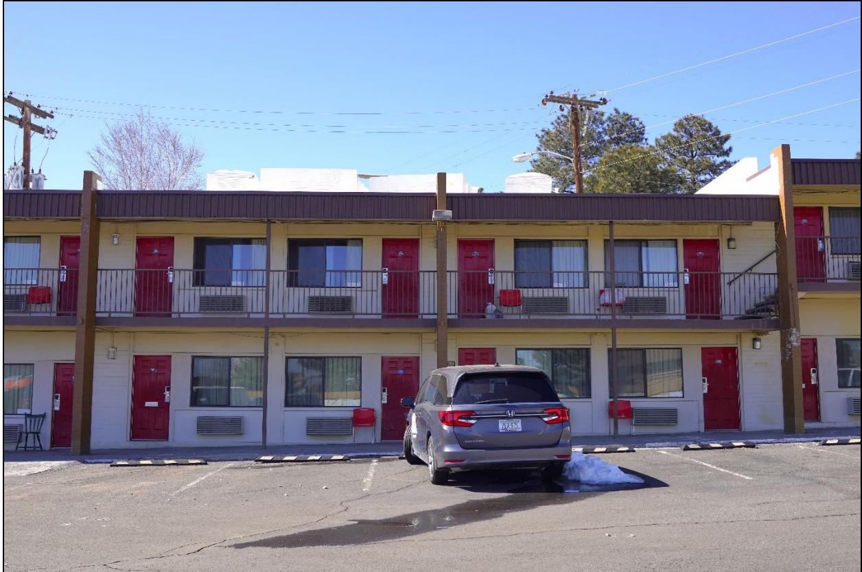
Figure 26. Photo of motel rooms in Building 1, facing west-northwest.
