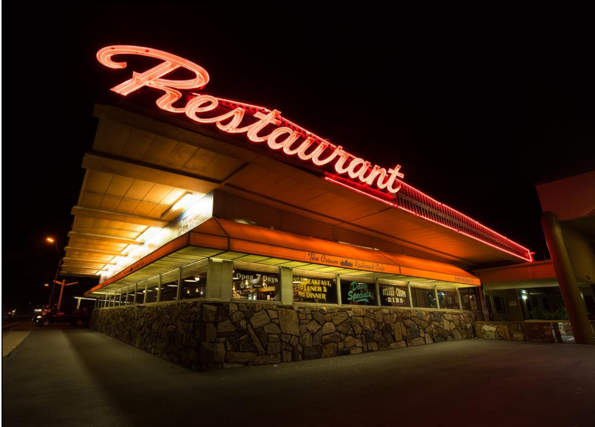
Figure 36. Pre 2024 photo of the Crown Railroad Café, photo credit Austin Corbett.
