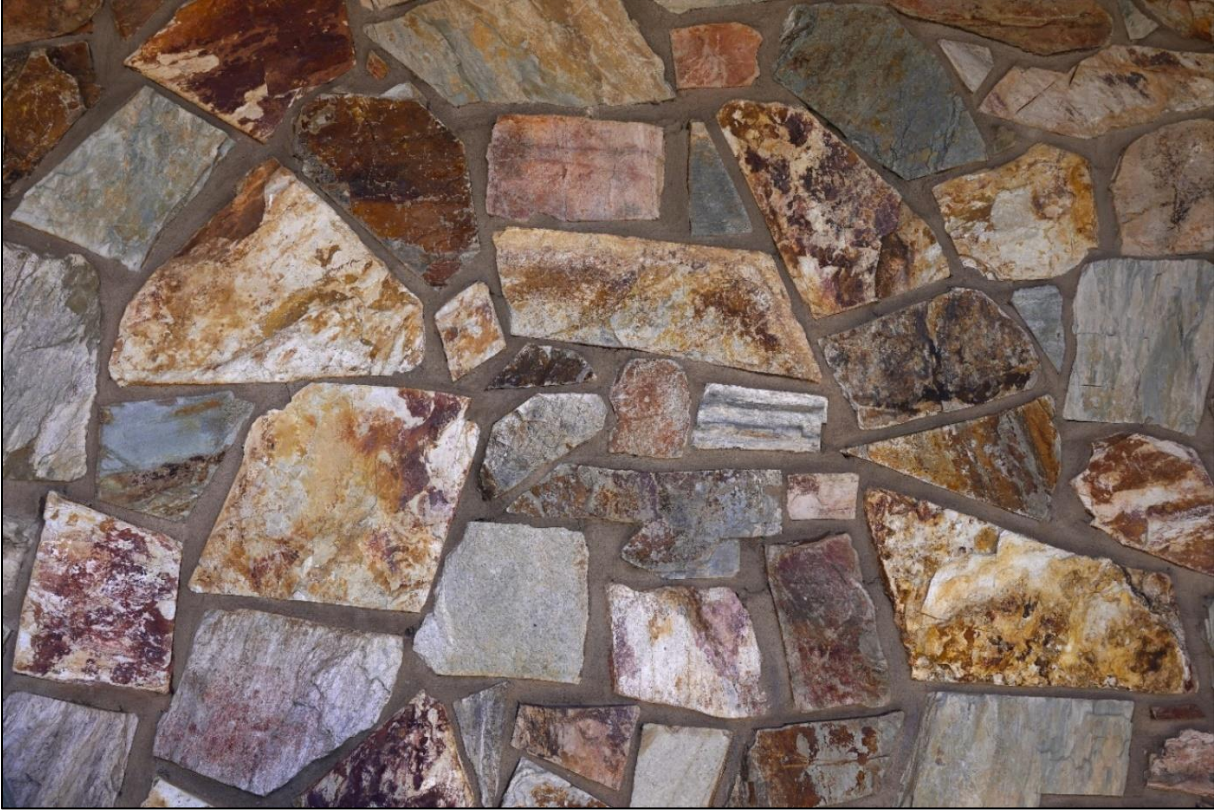
Figure 34. Photo of stone cladding.
