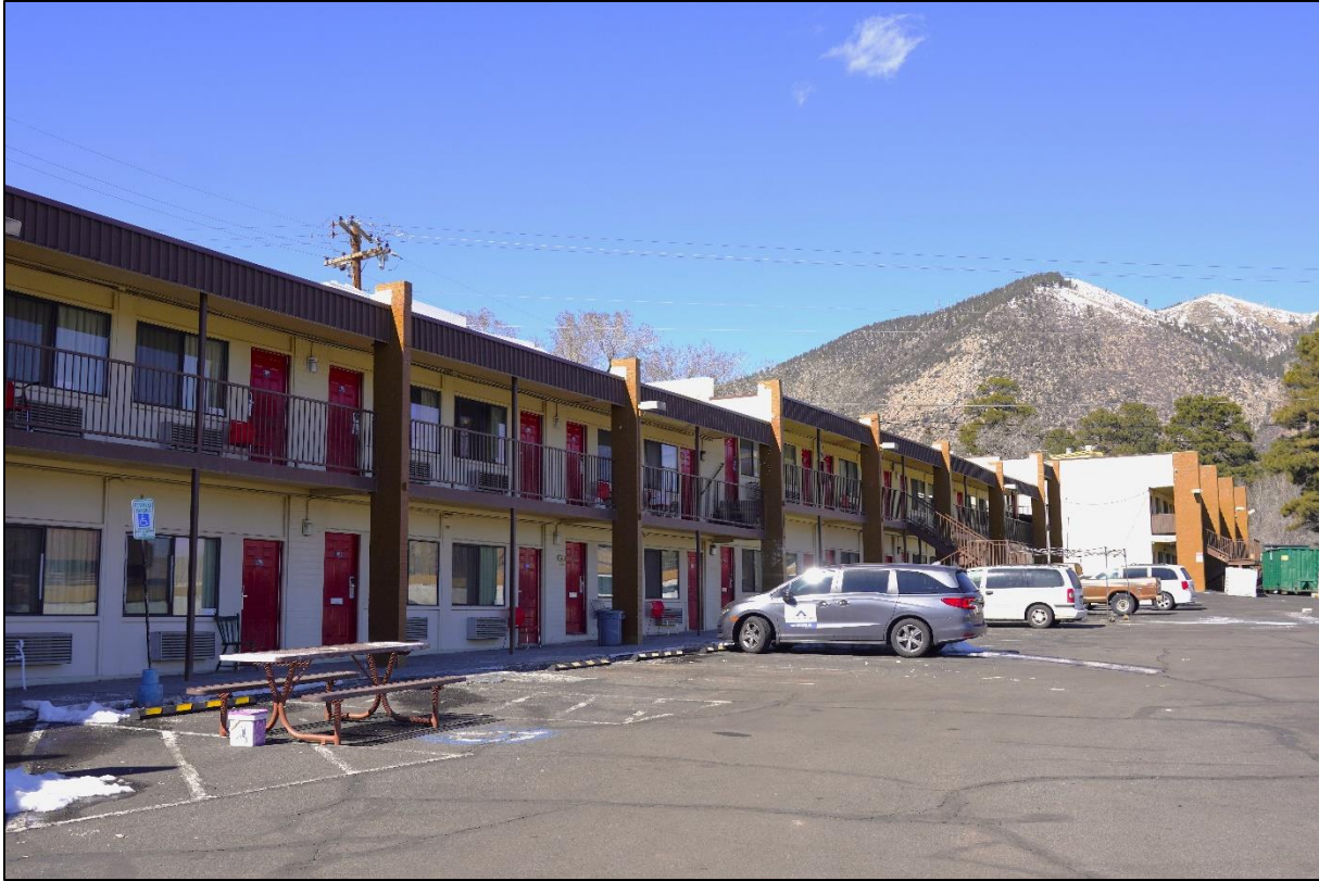
Figure 25. Photo of Building 1, facing northwest.
