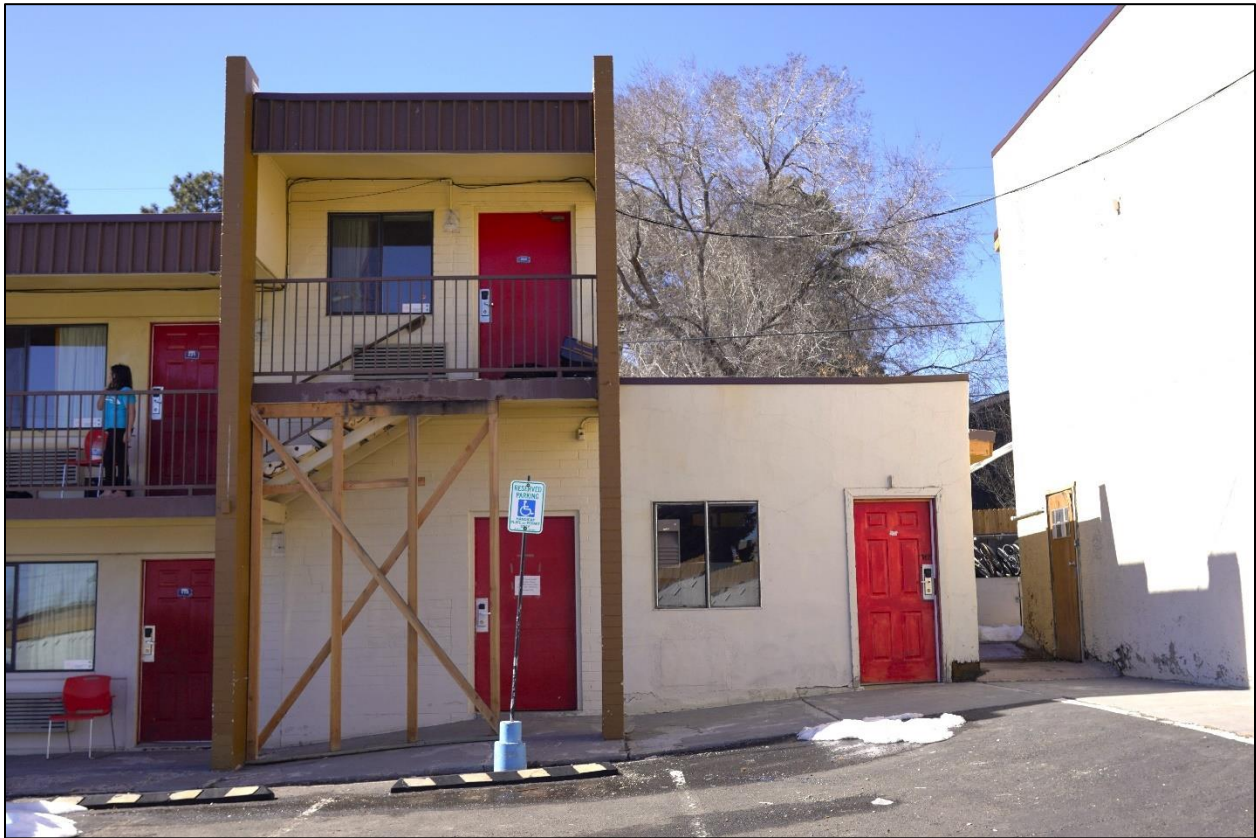
Figure 27. Photo of Building 1 1967 endcap, facing west-northwest.
