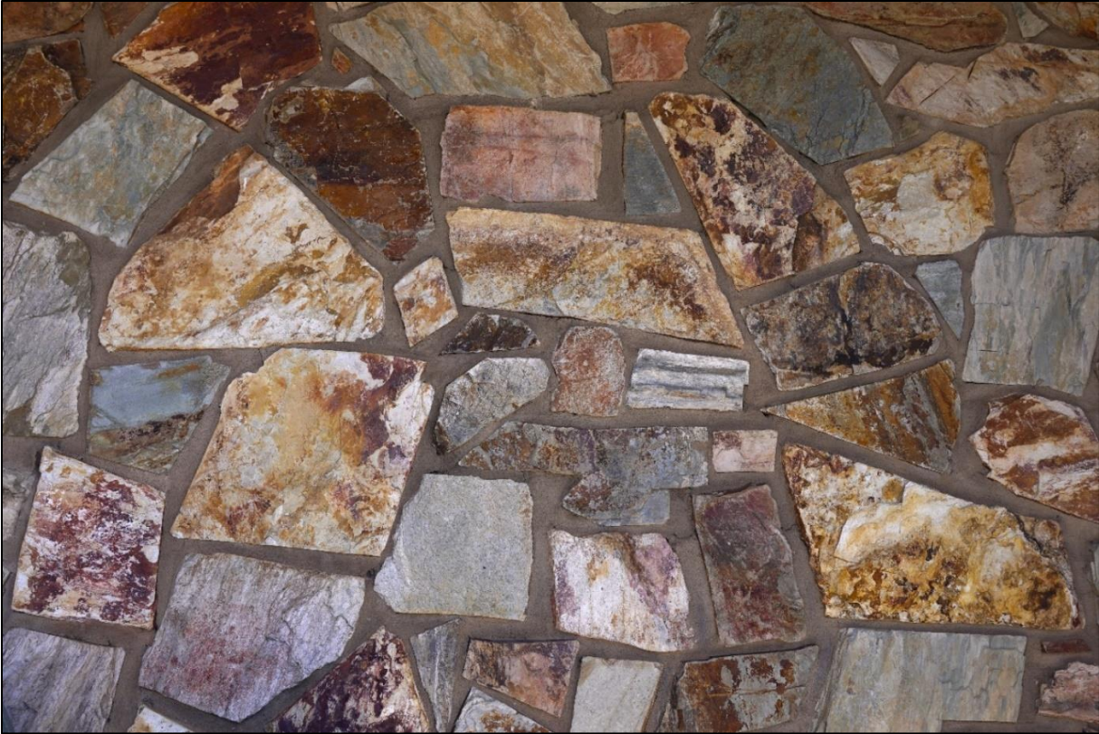
Figure 34. Photo of stone cladding.
