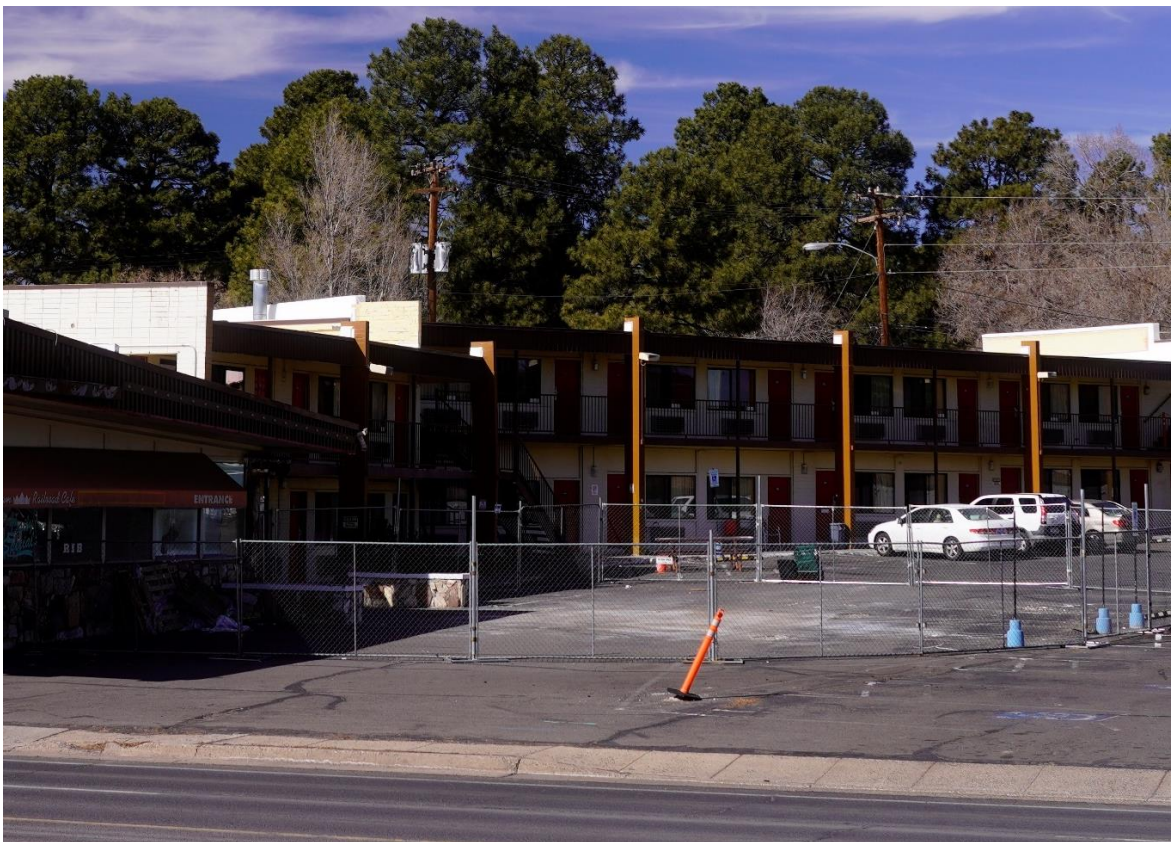
Figure 23. 2025 photo of porte cochere.
