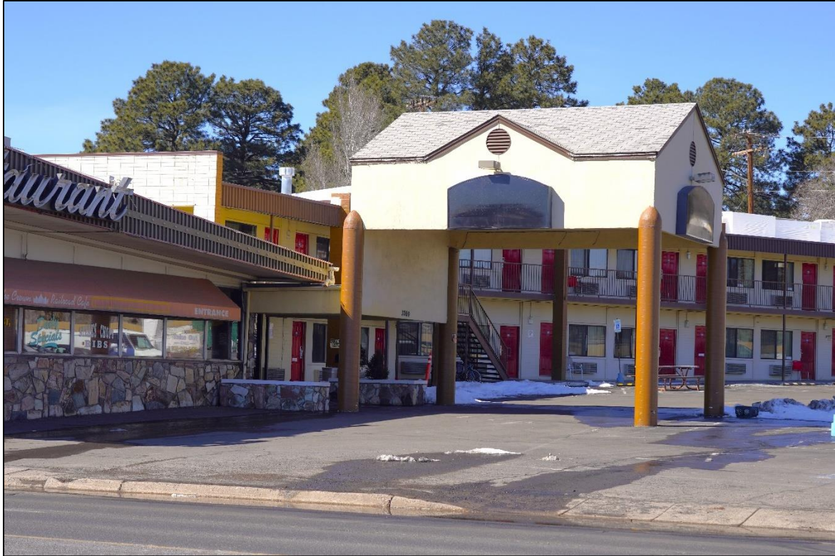
Figure 22. 2024 photo of porte cochere.
