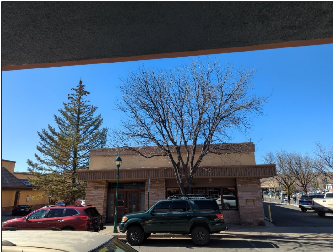
Photograph 1. Photograph of 123 North Leroux Street showing the eastern face of the building, facing west across Leroux Street.
