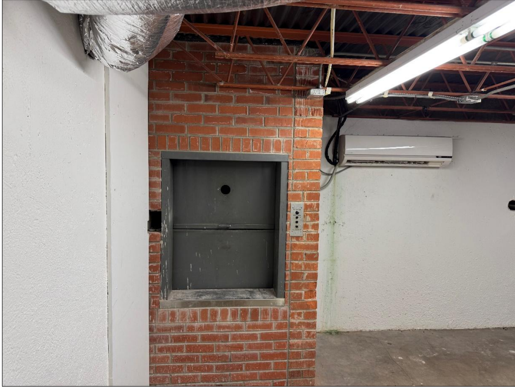
Photograph 6. A Sedgwick dumbwaiter located in the basement server room of 123 N. Leroux. The dumbwaiter was likely used during the property's existence as a bank, but remodeling has removed all other access points.
