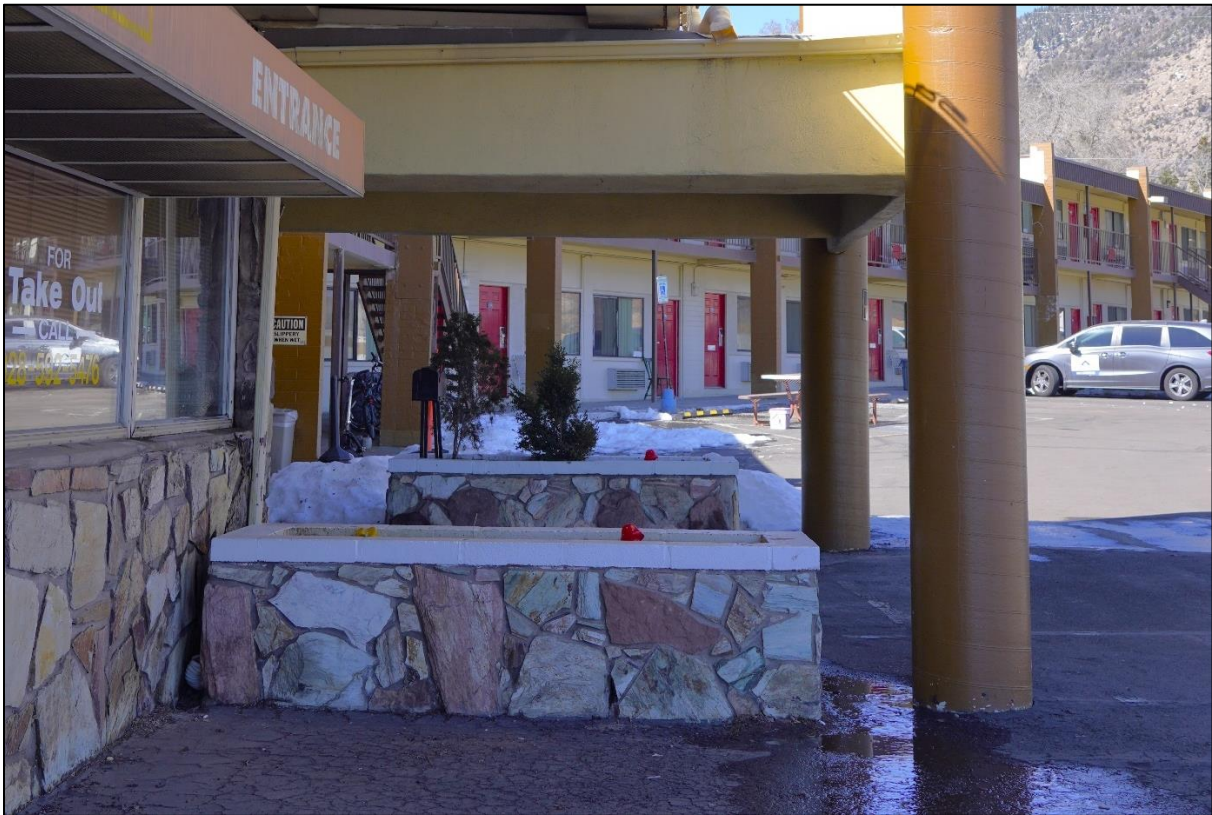
Figure 33. 2023 photo of stone cladding and original porte cochere.
