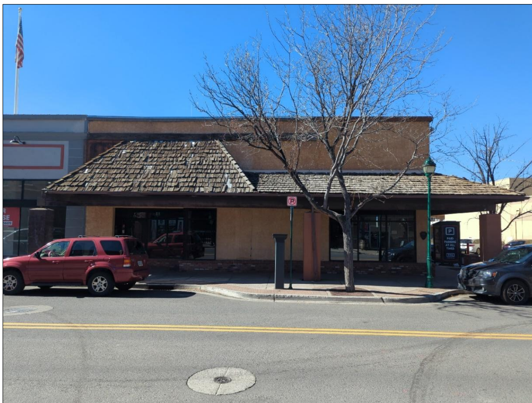
Photograph 1. The exterior of 111 N Leroux Street, facing west, no parking sign roughly marks the beginning of the 1994 additions, which extends to north.
