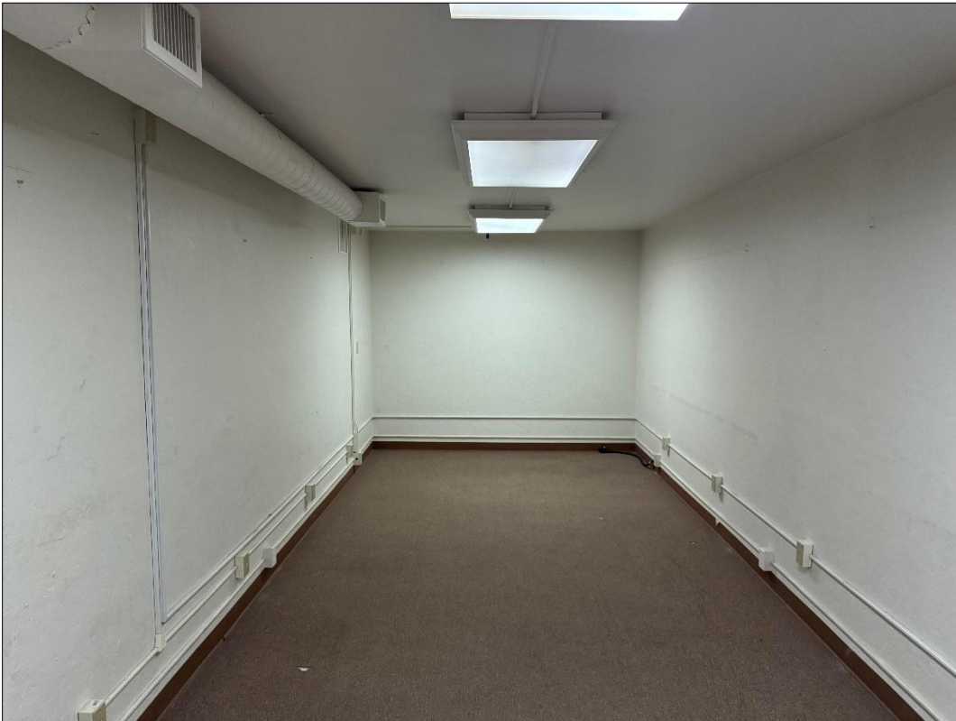
Photograph 5. The "Doyle" vault room which was possibly utilized as an office or storage space, facing west from the doorway.
