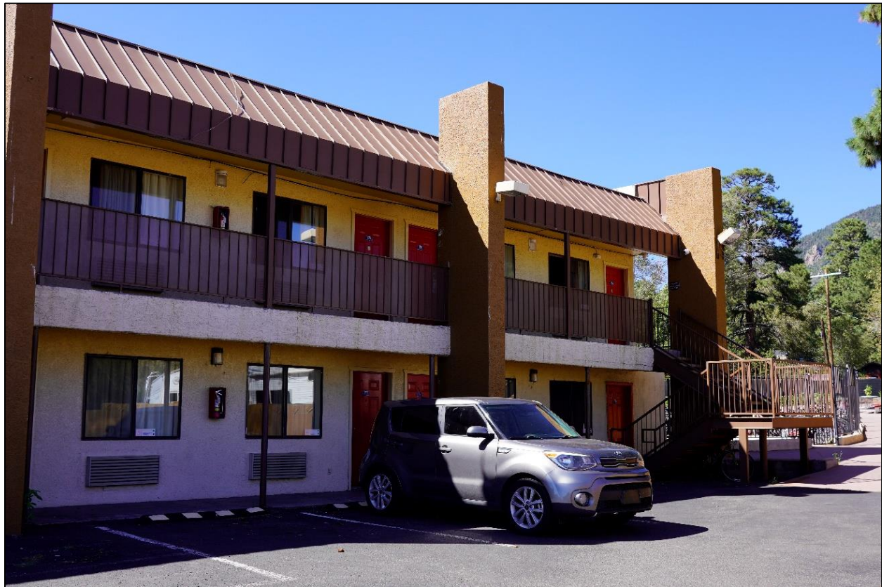
Figure 29. Photo of Building 2, facing northwest.
