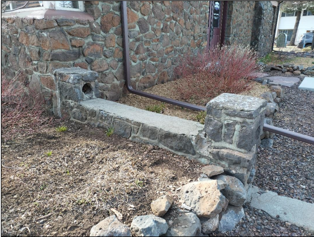
Photograph 3: West elevation extending wall
