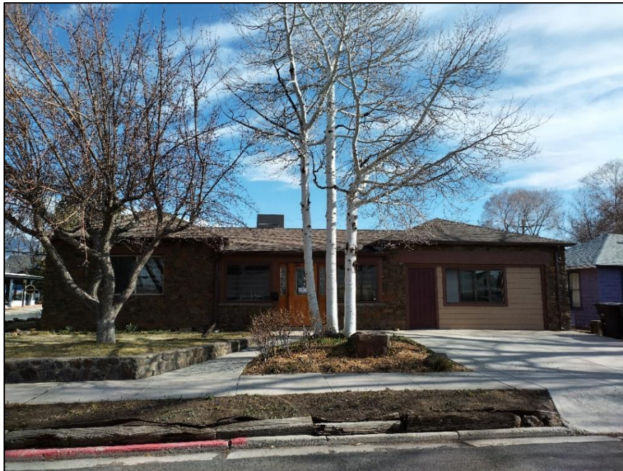
Photograph 1: South Elevation of Property showing original entryway from West Elm
