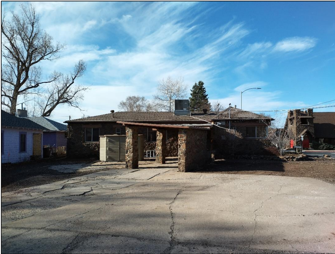
Photograph 2: North Elevation of Property showing modified outbuilding attachment
