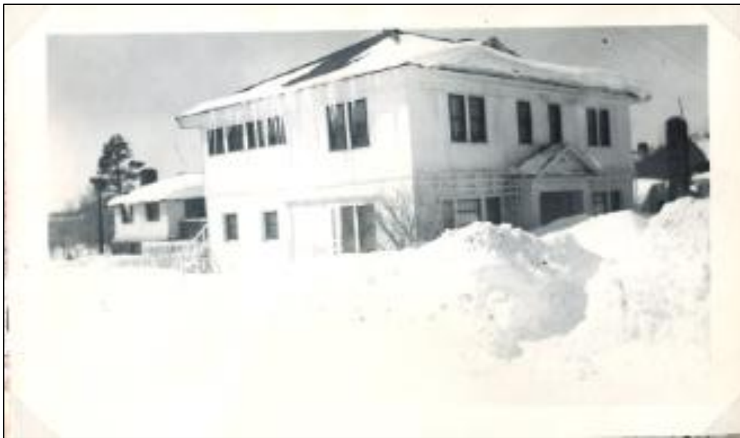
Photograph 1: Photograph of 23 E. Fine Avenue (1940s to 1950s) from San Francisco Street
