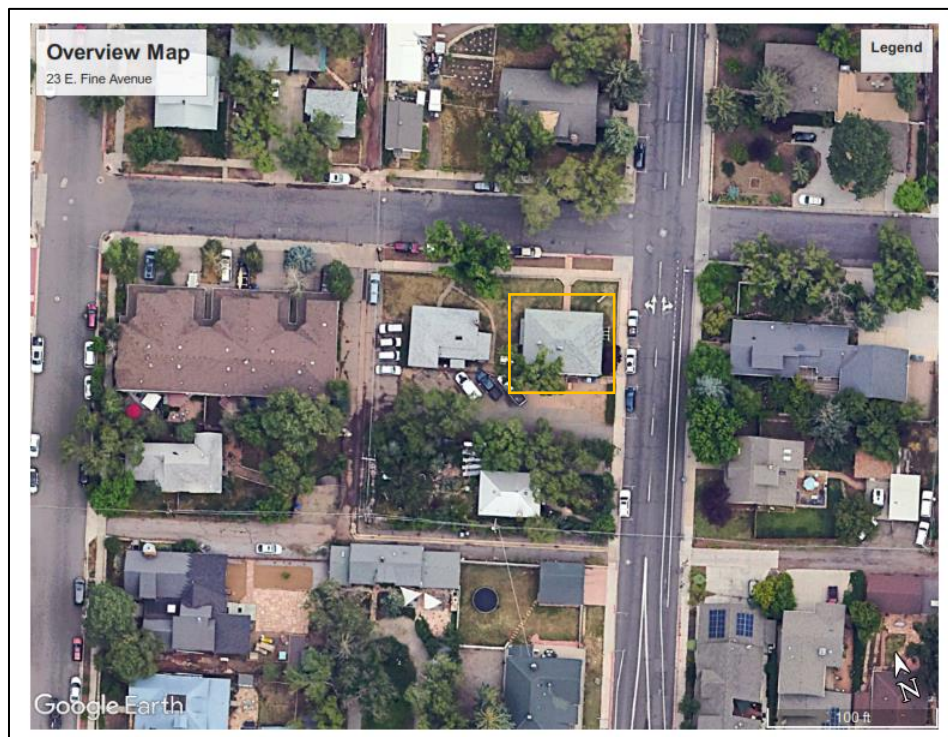
Figure 1: Overview map showing the Yaeger House (23 E. Fine Avenue) within orange square
