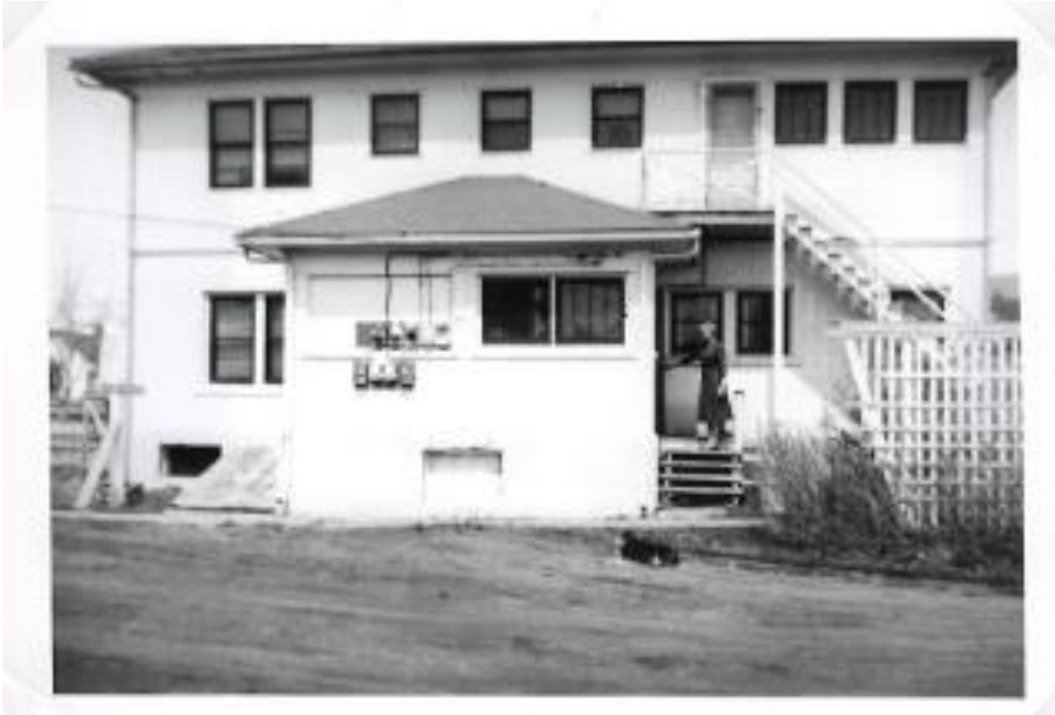
Photograph 2: Southern aspect of house circa 1940s
