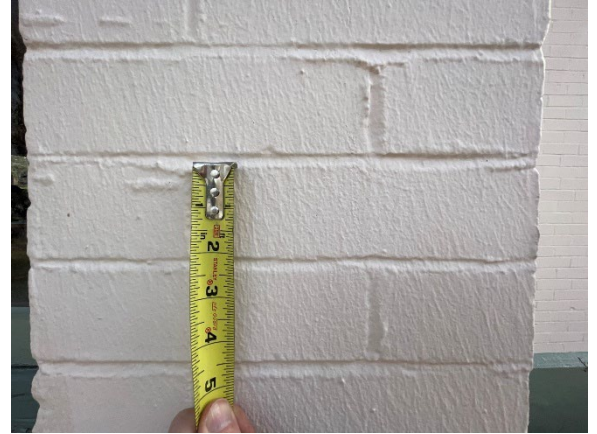
Photograph 4 – Typical Existing Brick Masonry
