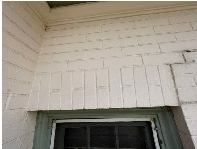
Photograph 5 - Existing "Flat Arch" Brick Masonry
