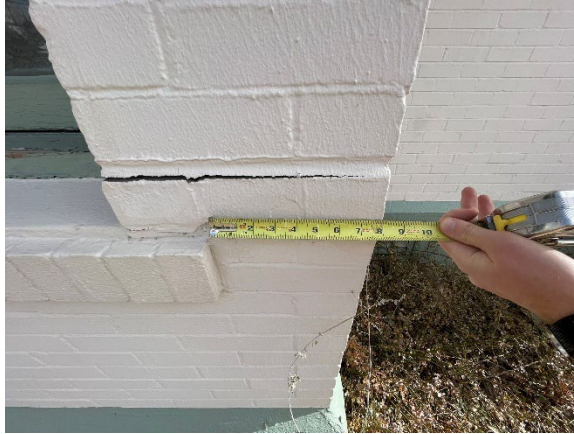
Photograph 3 – Typical Existing Brick Masonry
