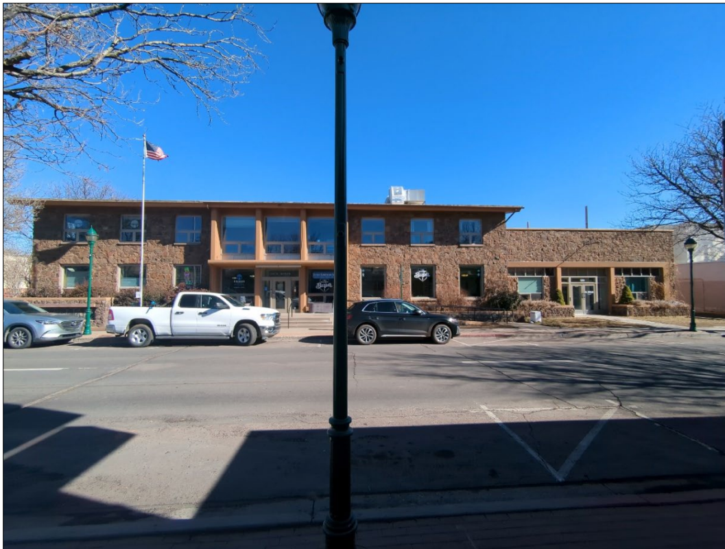
Photograph 2. West elevation of the studied building at 19 W Birch Ave, the City Hall and fire department portions of the building are visible.
