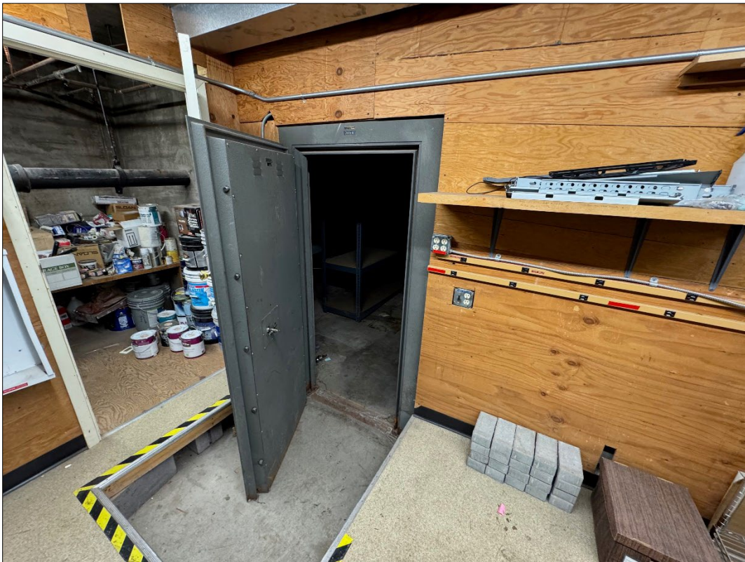
Photograph 11. The basement vault room which was once used to hold city records and receipts.
