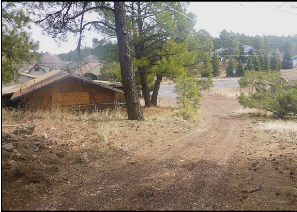
Figure A-14. West elevation and driveway of Unit 2; view facing southwest.
