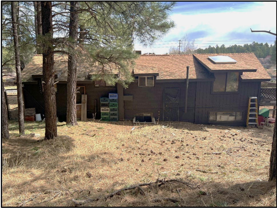
Figure A-4. West elevation of Unit 1; view facing east.
