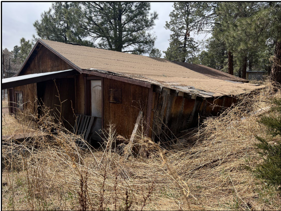
Figure A-10. North and east elevations of Unit 2; view facing southwest.
