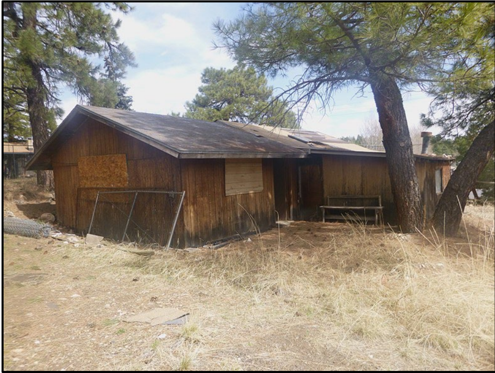
Figure A-12. South and west elevations of Unit 2; view facing northeast.
