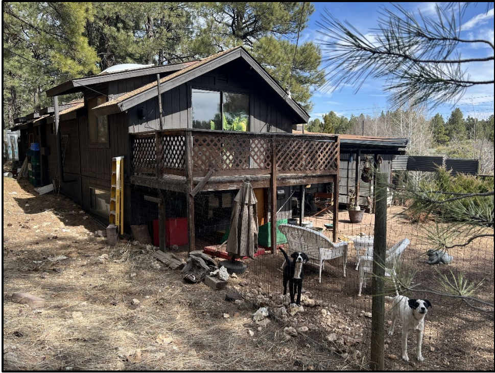
Figure A-3. South and west elevations of Unit 1; view facing northeast.
