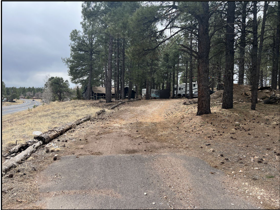
Figure A-8. Driveway of Unit 1; view facing southwest.
