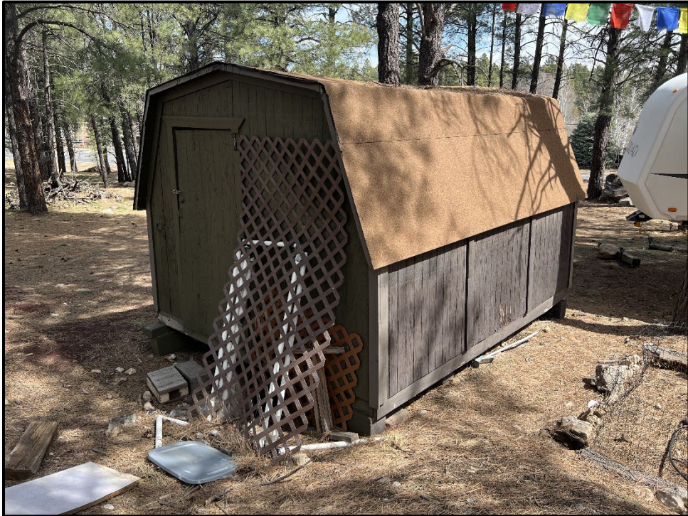
Figure A-6. Shed feature adjacent to Unit 1; view facing northeast.
