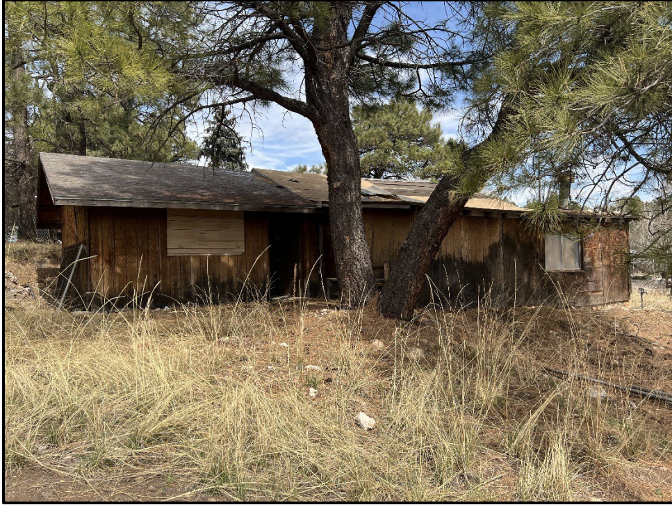
Figure A-11. South elevation of Unit 2; view facing north.
