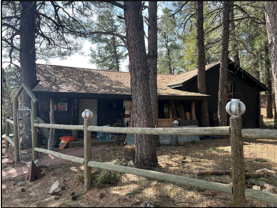
Figure A-1. North elevation (entrance) of Unit 1; view facing south.
