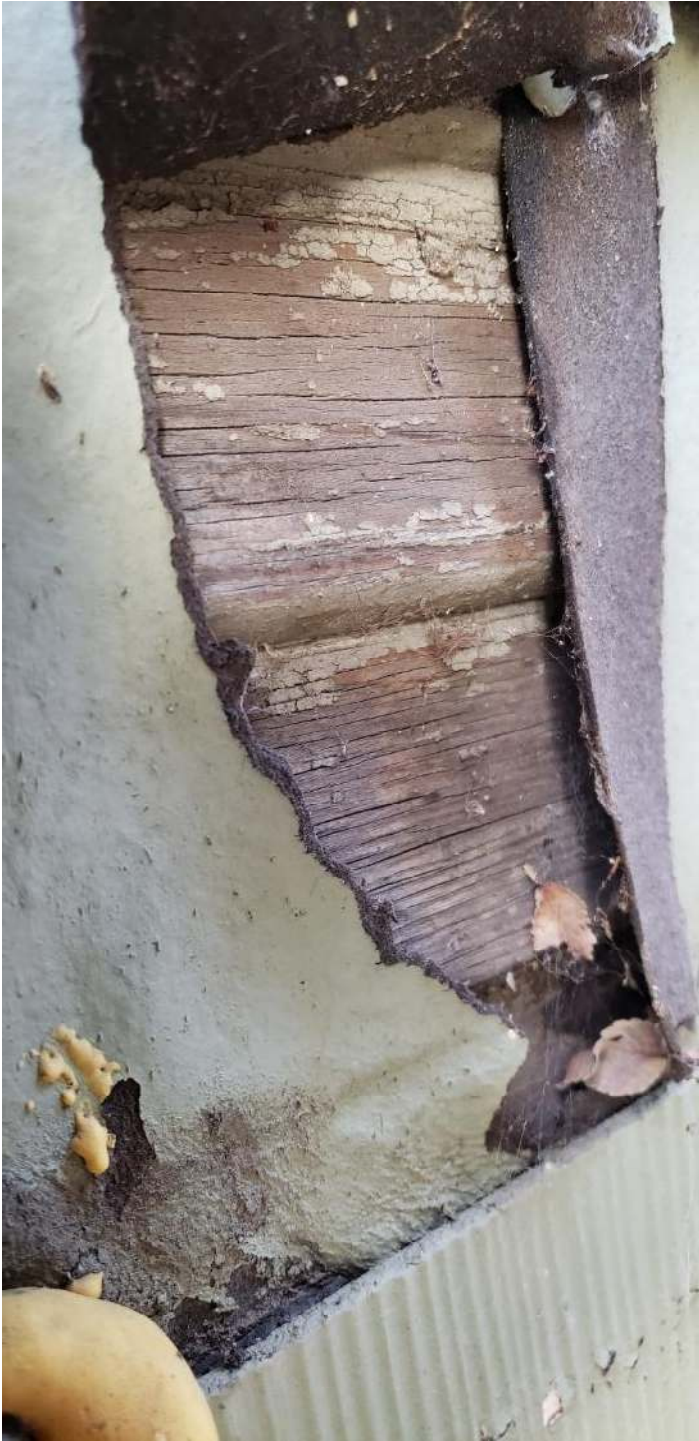
Photos 23–24. 418 E Birch Ave E façade detail of likely original clapboard siding under later Transite shingles facing NW (left), and detail of the clapboard siding on house's interior (what was the original N façade) facing SW (right).
