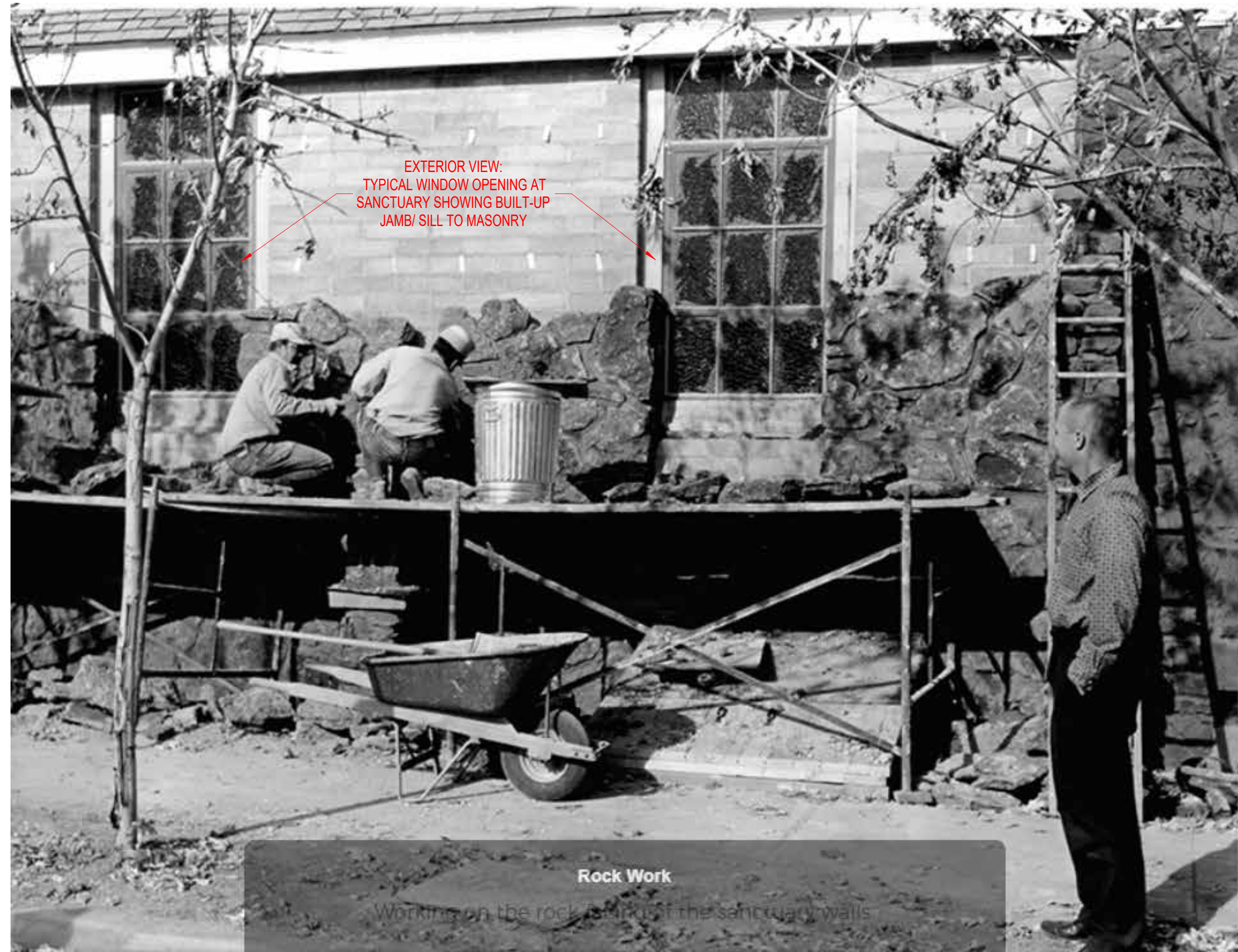
09 - HISTORICAL EXTERIOR - DURING CONSTRUCTION
