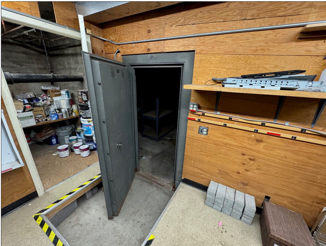
Photograph 12. The basement vault room which was once used to hold city records and receipts.
