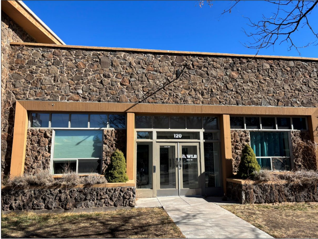
Photograph 5. East facing photograph showing the entryway to southern portion of the building which once housed the fire department.
