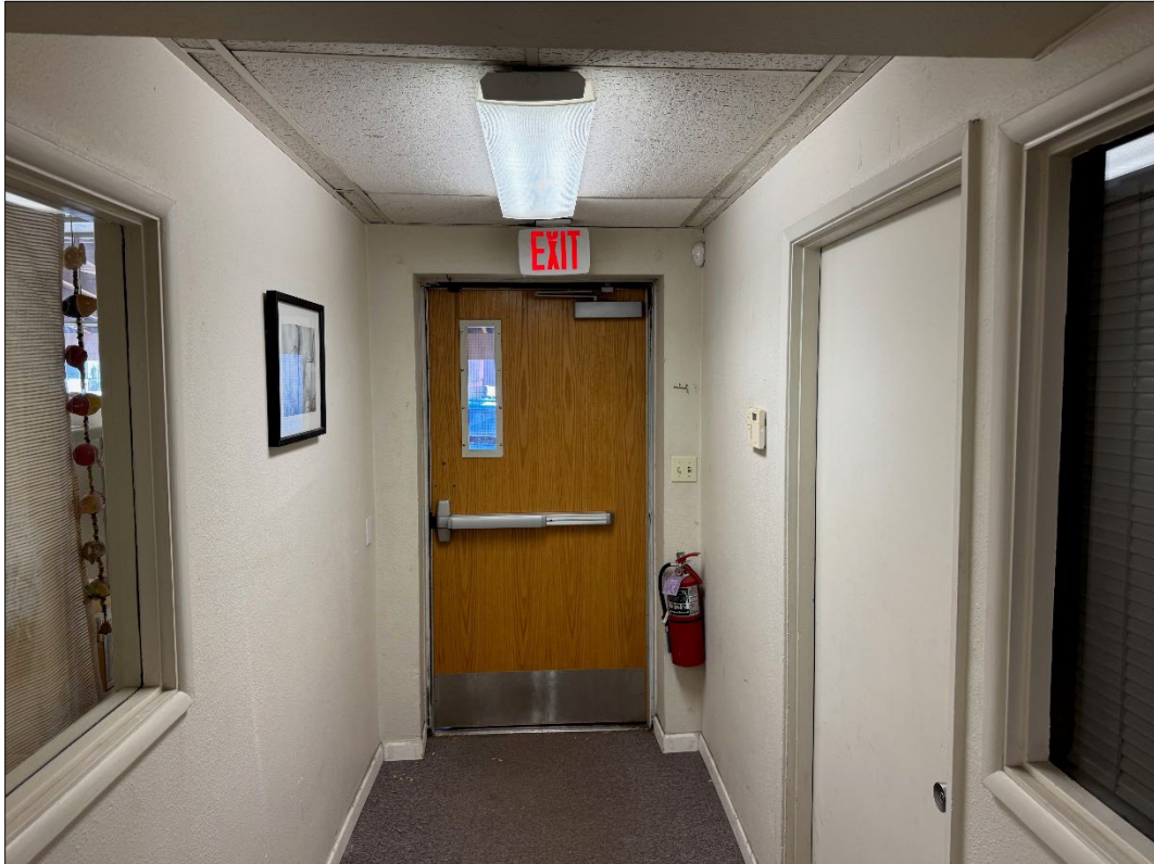
Photograph 14. South facing photograph showing the south entrance to the former Police Department.
