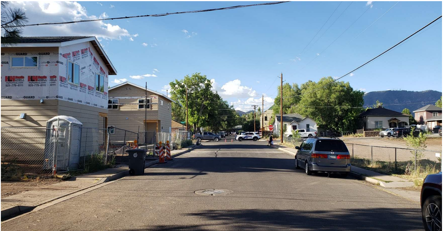
Photos 13–14. 415 W Tucson Ave rear house to NE from alley with fencing of 205 S Park St location in left background ( top ) and overview from middle of Park St to N showing 205 S Park St/405 W Tucson Ave lot and, left to right, 123 S Park, 324 W Tucson, 318 W Tucson in background on N side of W Tucson ( bottom ).
