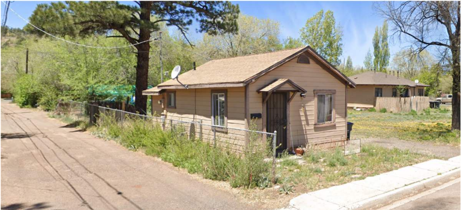
Photos 1–2. 205 S Park St house in left background and facing 405/407 W Tucson Ave from N side of Tucson to SSW ( top ) and front/E and S façades to NW from Park St with 407 W Tucson in right background ( bottom ).
