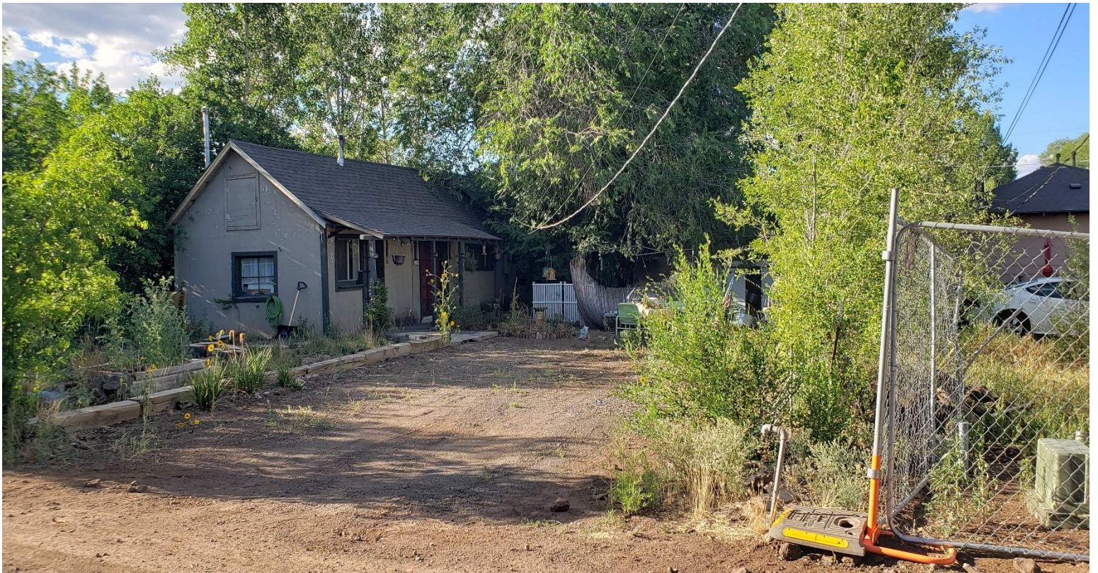
Photos 11–12. 205 S Park St location to NE showing new construction, outbuilding, and 407 W Tucson in left background ( top ) and 409 W Tucson Ave to NW showing S end of modified historic house and 407 W Tucson in right background ( bottom )
