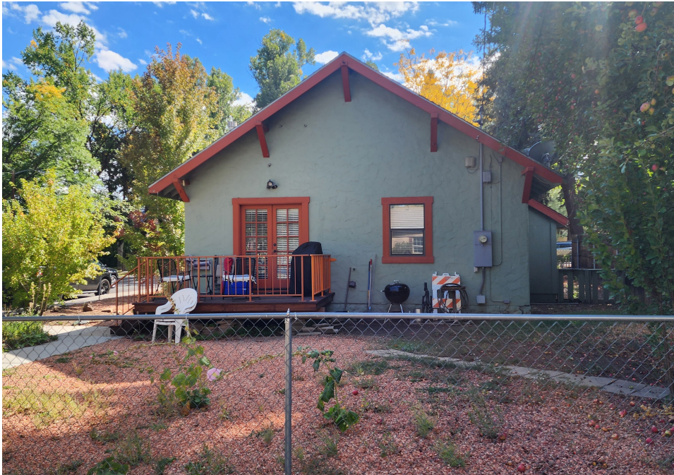
SUBJECT SITE - 402 W BIRCH AVE. - NORTH SIDE
