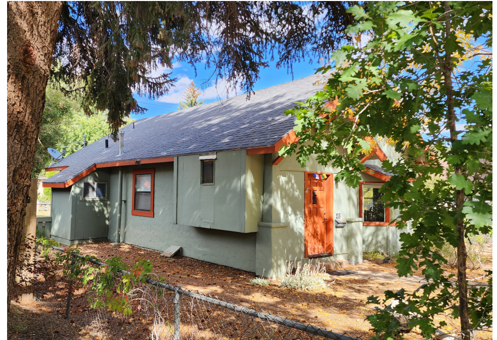
SUBJECT SITE - 402 W BIRCH AVE. - WEST SIDE
