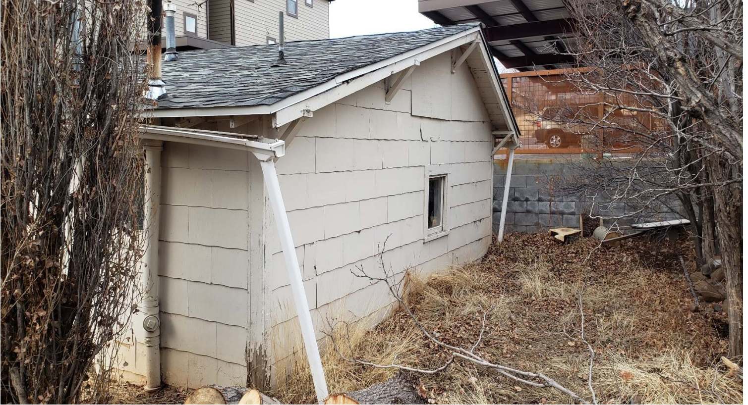
Photos 15–16. 314 N Beaver St Unit 5 front/W façade (top) and rear/E façade facing NW (bottom).
