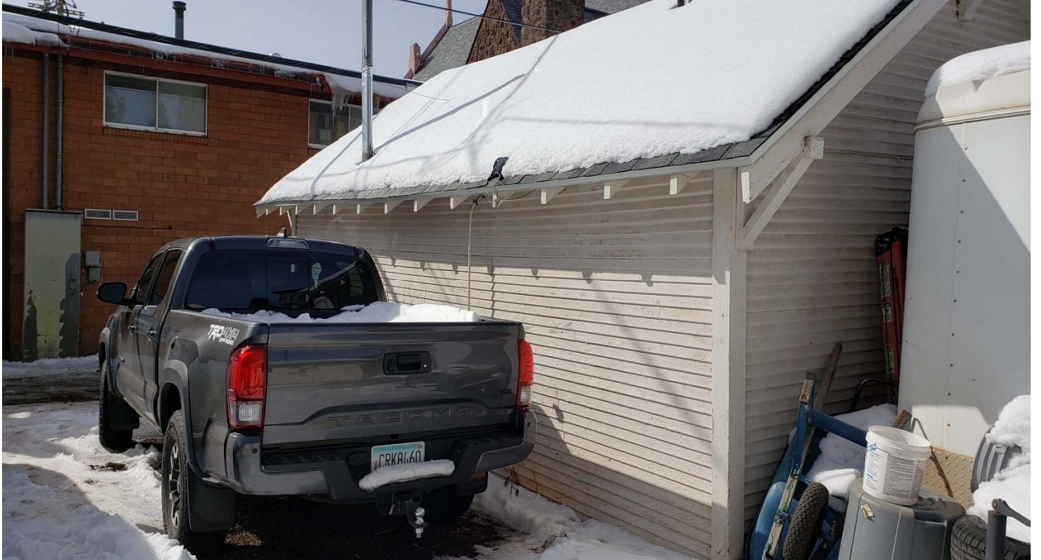
Photos 7–8. 314 N Beaver St Unit 4 W façade to SE (top) and E façade/NE corner to SW (bottom).
