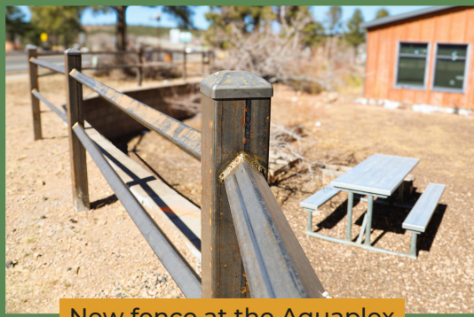
New fence at the Aquaplex
