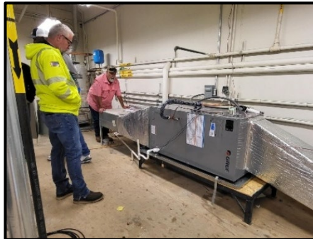
Photos: New cold-climate heat pumps installed at Fire Station 1 (left) and the Fire Training Center (right) and inspected by Facilities staff.
