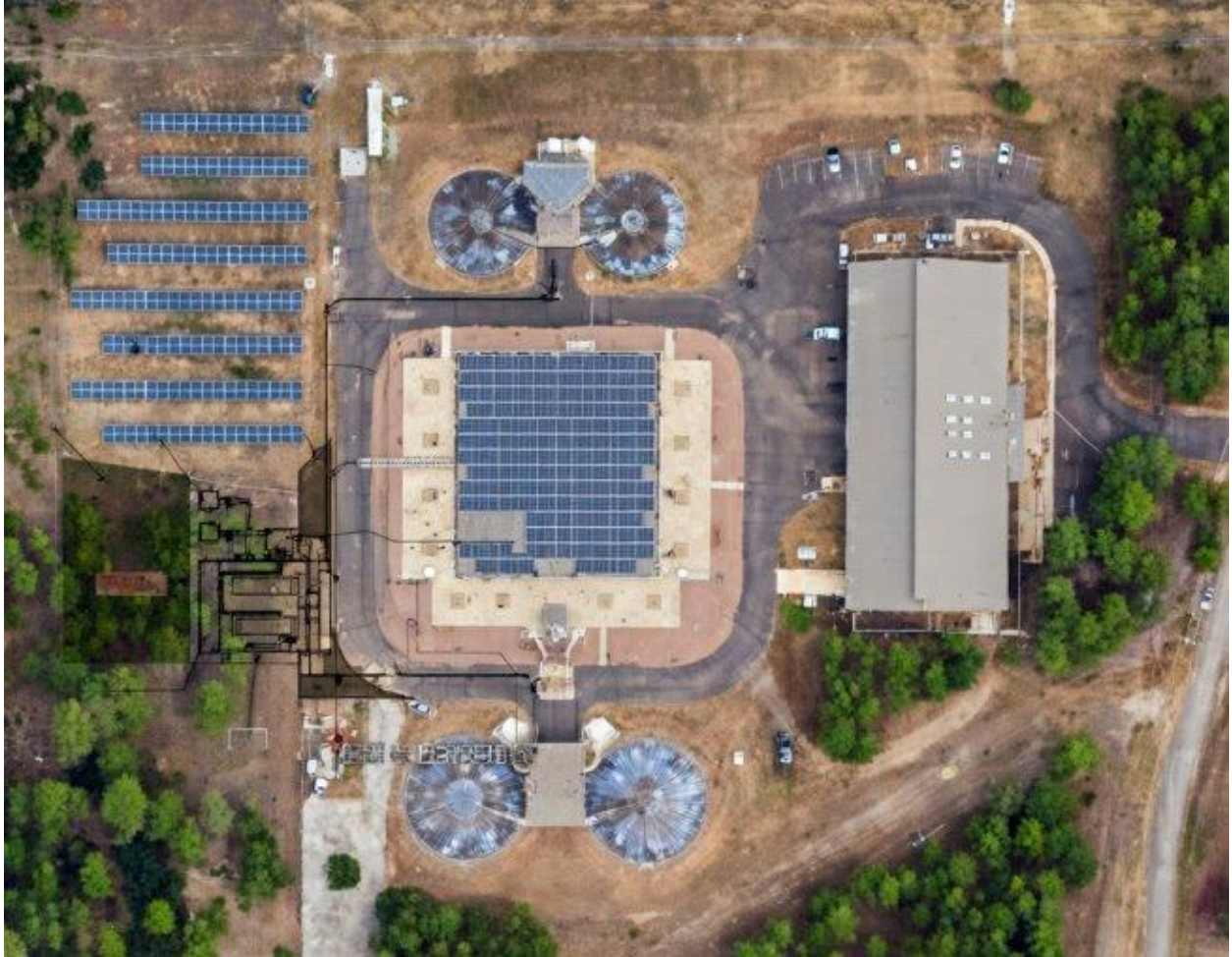
Rio de Flag Water Reclamation Plant with Solids Handling Facility Footprint
