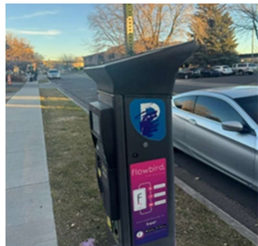
Figure 2. Vandalized Pay Station
