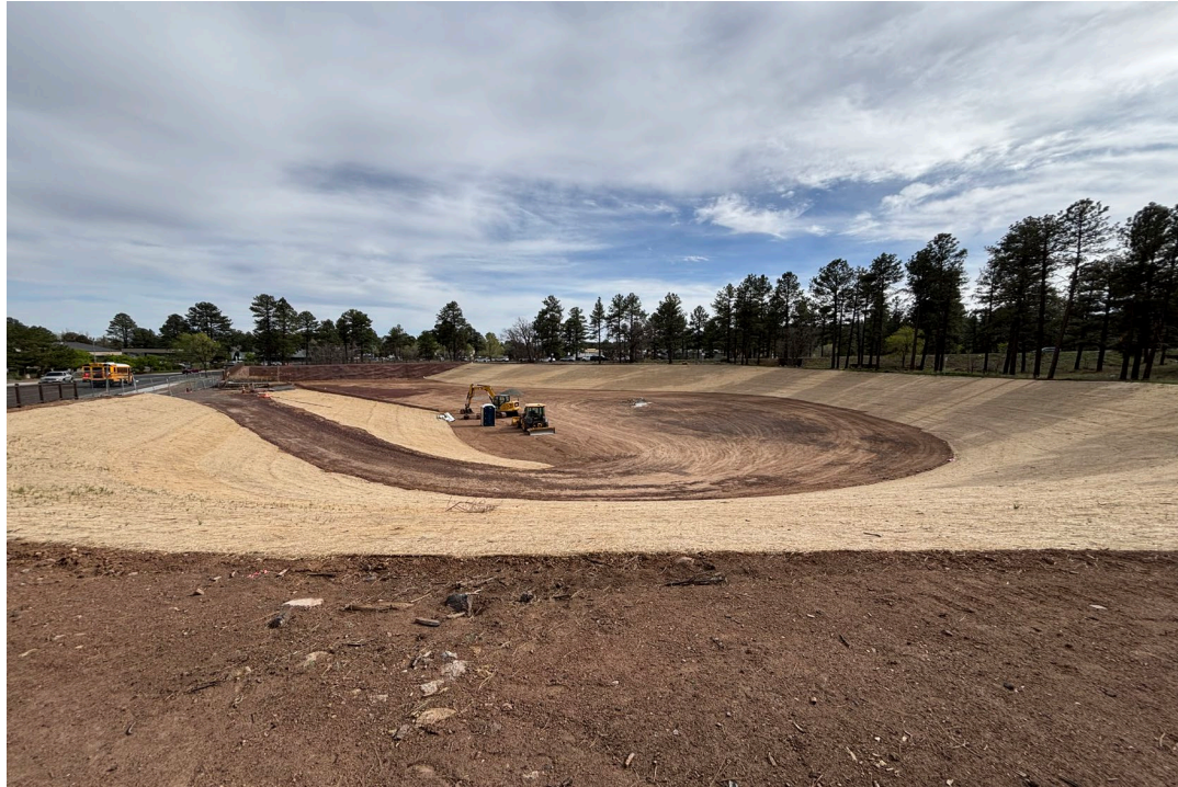
"The Wedge" Detention Basin
