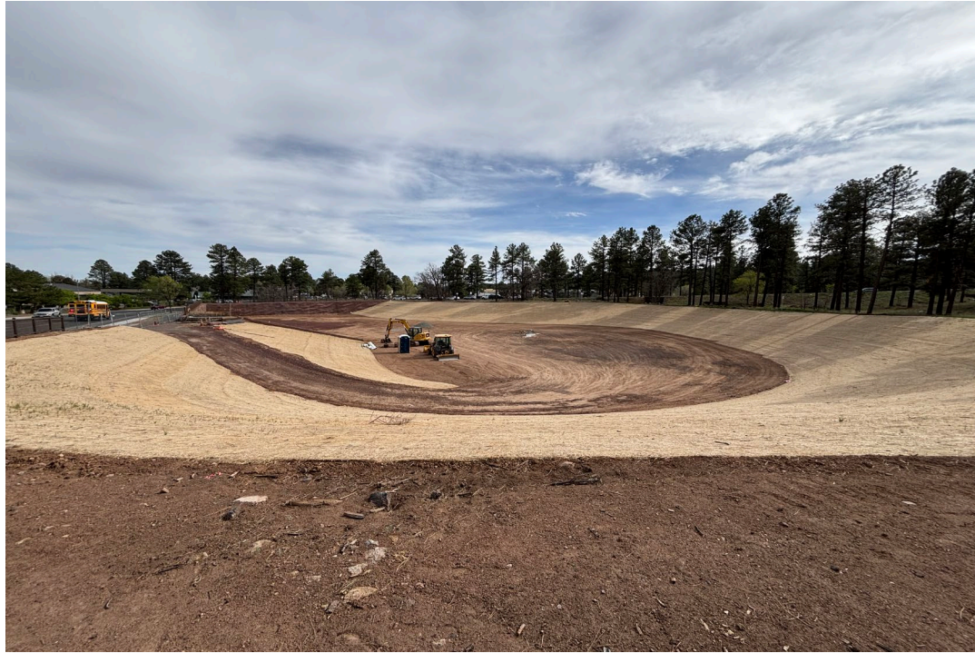
"The Wedge" Detention Basin
