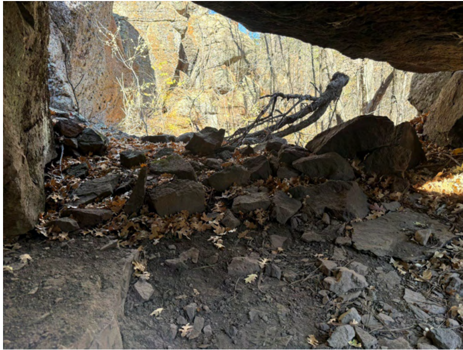
Figure 12 Feature One (F1) dry-laid masonry wall at Sanctuary Four, view east.
